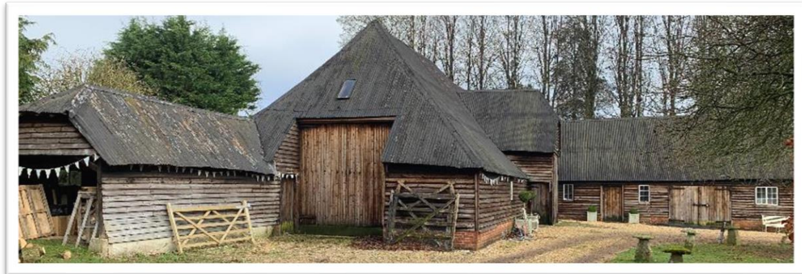
Figure 5: Old asbestos roofed barn in the north of the site.
