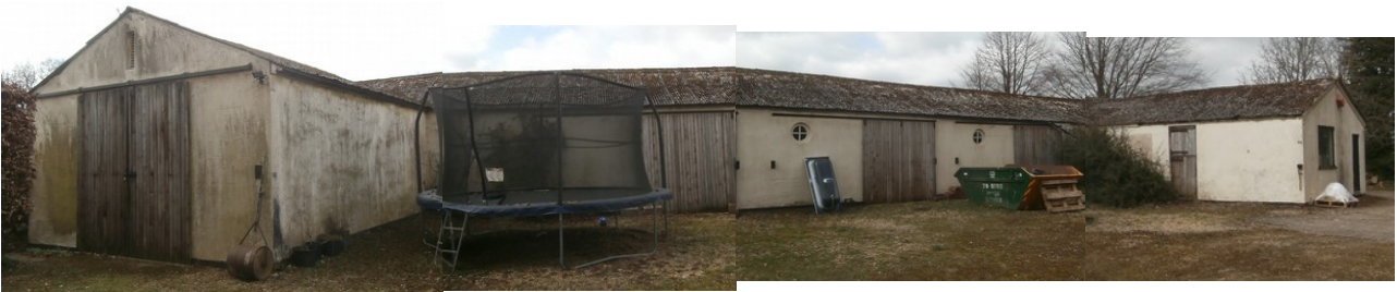
Recently demolished block
