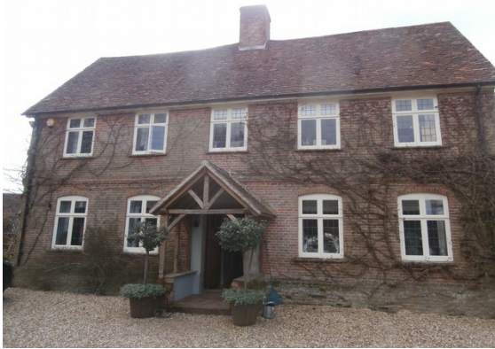
Manor Farmhouse – north elevation
