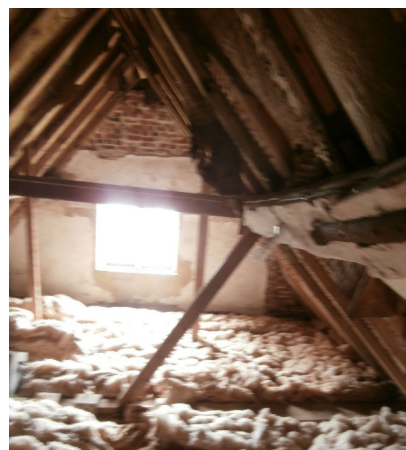
Former room in the roof
