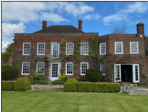
Figure 4 – south elevation of the main house
