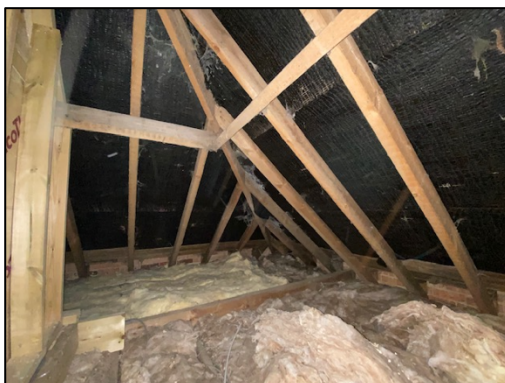
Figure 6 – roof void beneath the western hip end
