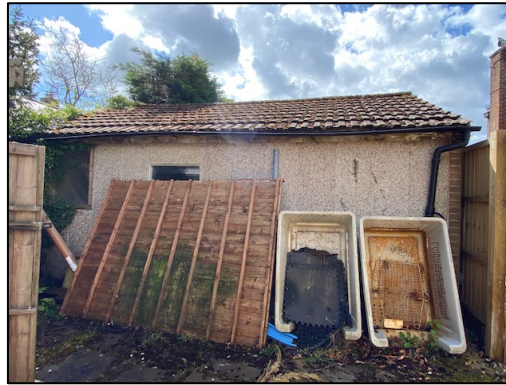
Figure 8 – northern elevation of the outbuilding
