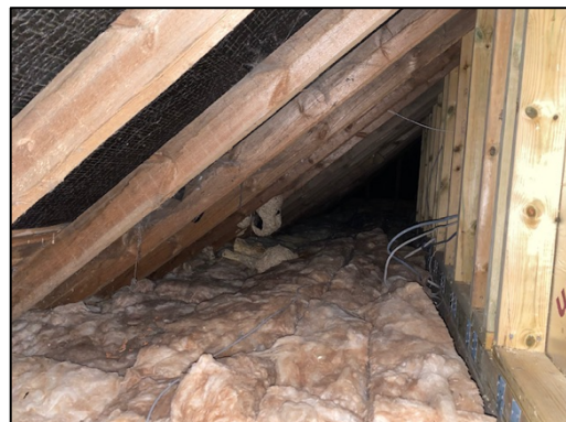
Figure 7 – northern area of the roof void
