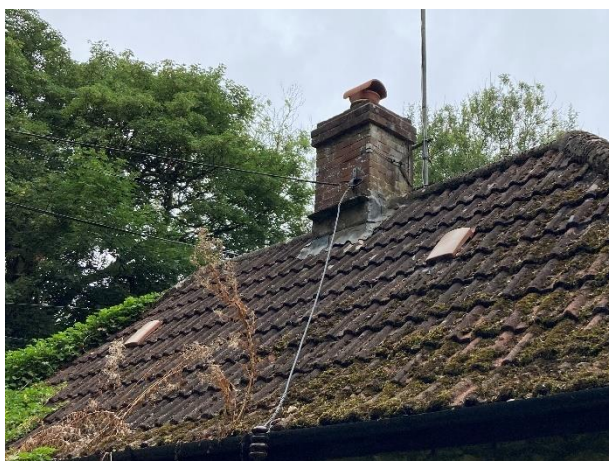
Photo 11, "Gaps between the chimney and lead flashing"
