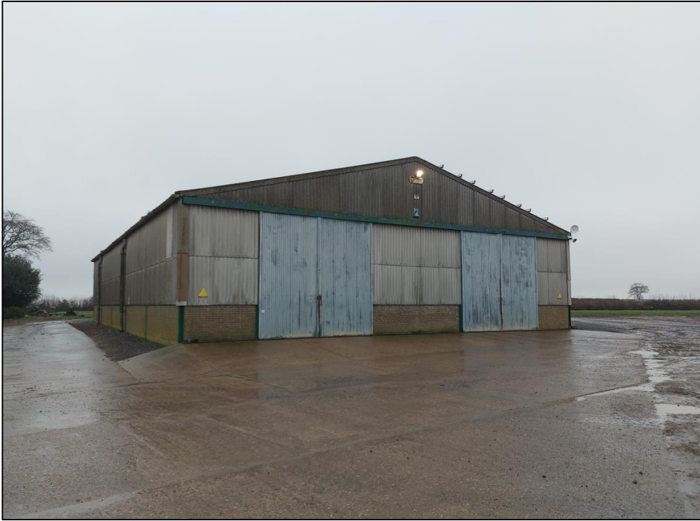
Photograph 1: View looking east towards western elevation of agricultural building to be extended.
