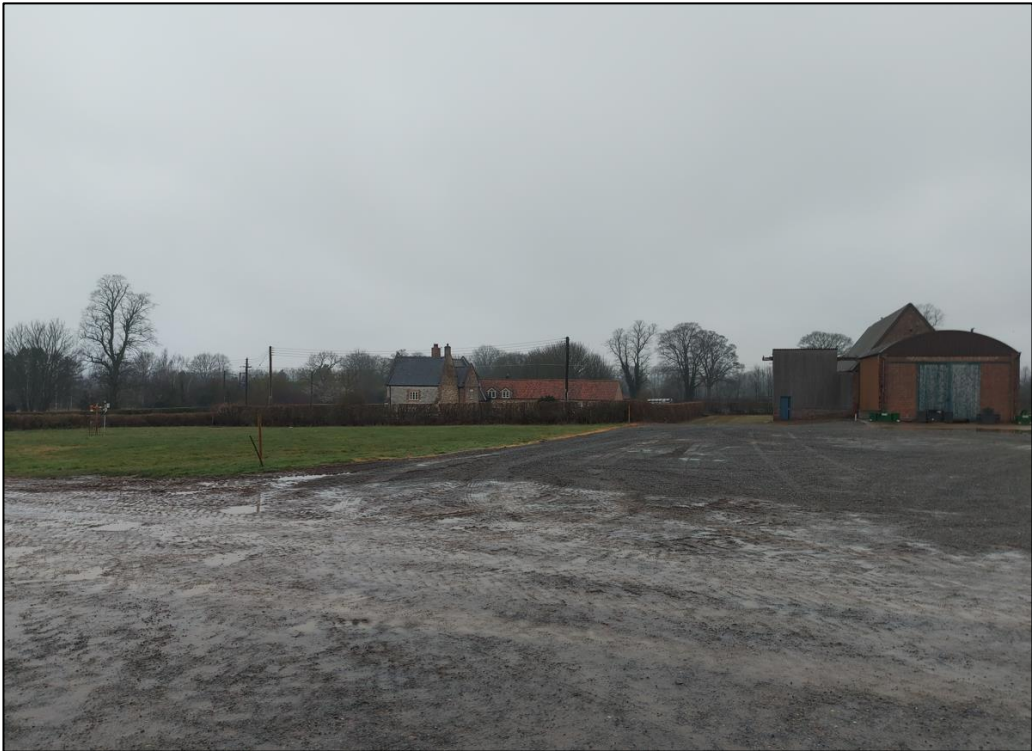
Photograph 2: View looking north across farmyard towards Hill Farm House.
