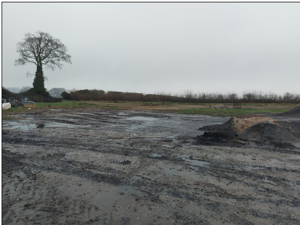
Photograph 6: View looking east across site of new extension.
