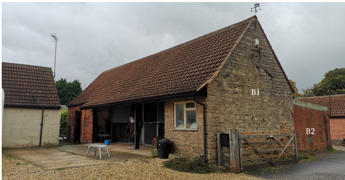
Figure 09 – Photo from southeast corner of site
