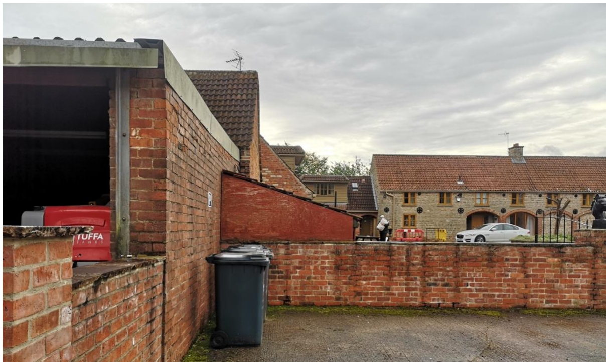
Figure 06 – Looking towards The Stables and converted Coach House (Photo taken from proposed north elevation looking south)
