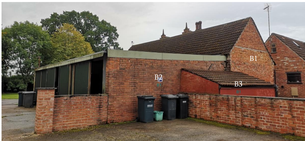
Figure 10 – Photo from northwest corner of site
