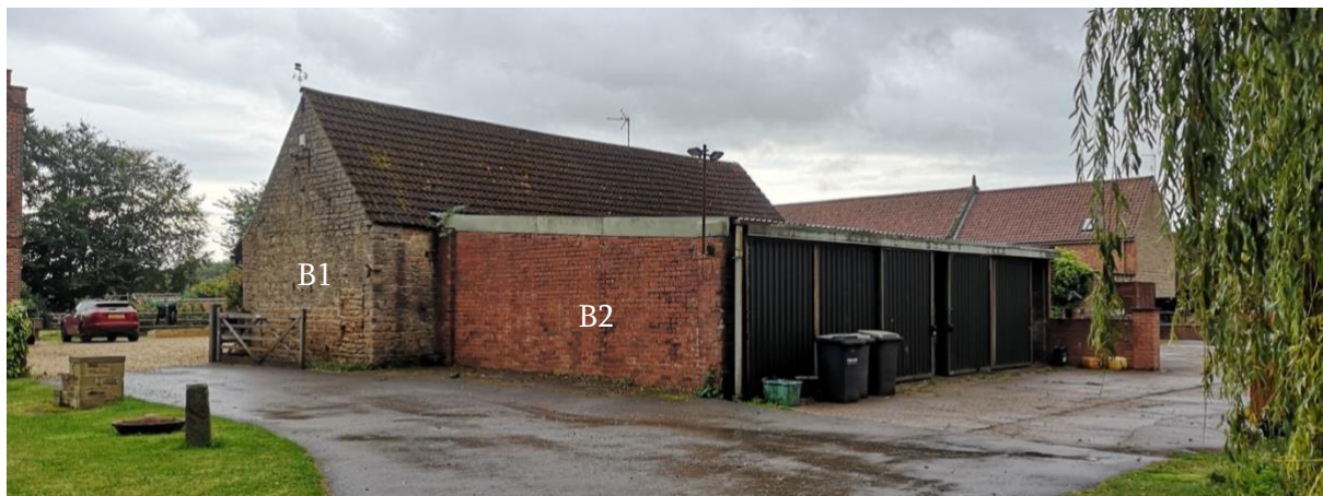
Figure 08 – Photo from access road, northeast corner of site
