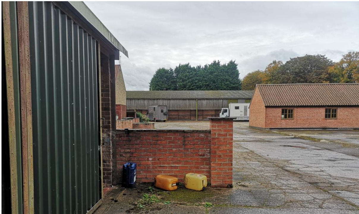
Figure 05 – Looking towards The Stables and converted Coach House (Photo taken from proposed north elevation looking west)
