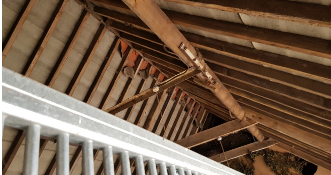
Figure 1 Rafters, purlins, trusses and splice
