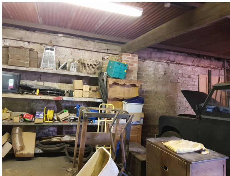
Figure 6 North wall seen from the garage
