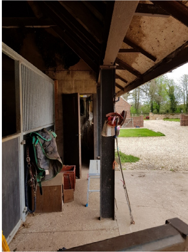
Figure 2 Steel arrangement in front (South) wall
