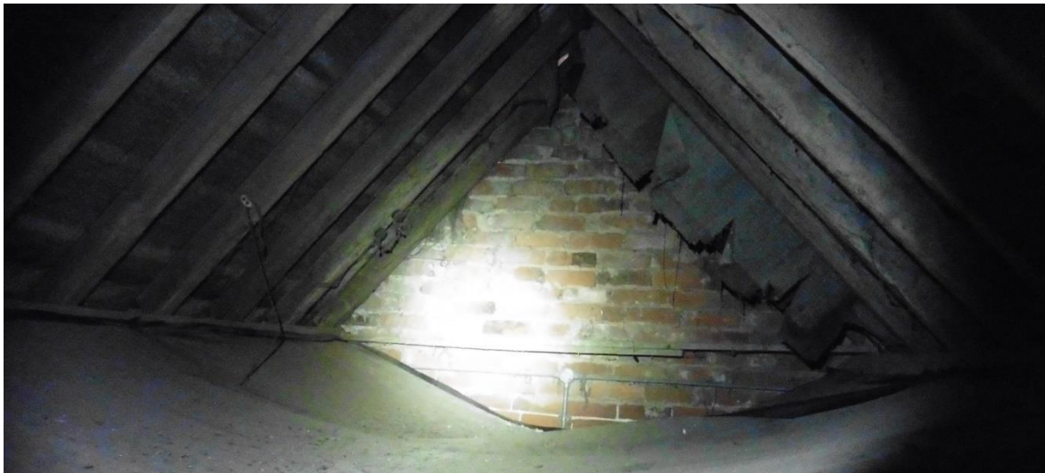
Photograph 4: Attic space at west end of traditional part of outbuilding
