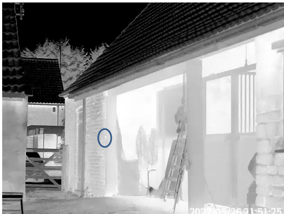
Photograph 10: South elevation of outbuilding at Abbeyfields farm with location of day roost of Soprano Pipistrelle indicated as identified during bat emergence and activity survey 26 th May 2022
