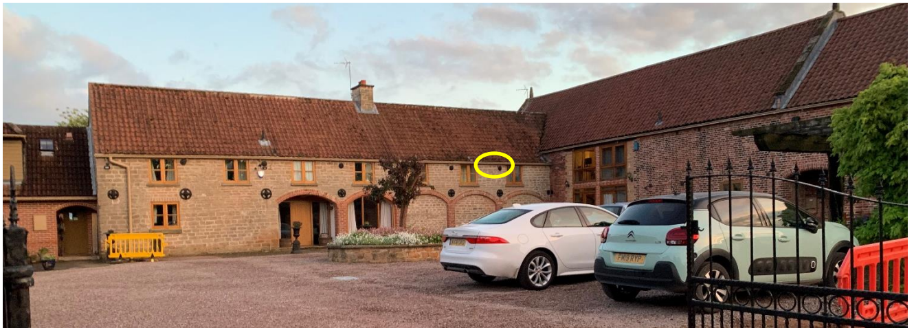
Photograph 11: North elevation of converted coach house and stables situated to the south west of the survey area with location of Common Pipistrelle maternity roost indicated as per bat emergence and activity survey 26 th May 2022
