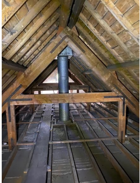
Fig. 13: Roof void with ventilation shaft
