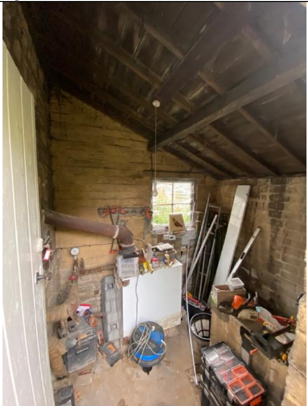
Fig. 15: Interior of lean-to at south elevation
