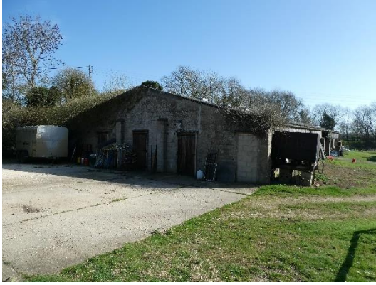
Photograph 1: Western elevation of the shed
