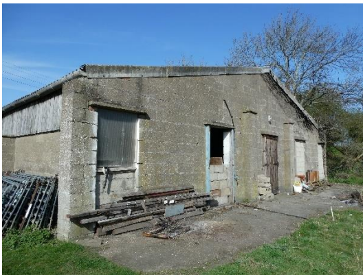
Photograph 3: Eastern elevation of the shed
