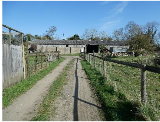
Photograph 14: Fencing along the western boundary
