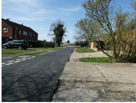
Photograph 17: Vicarage Lane to the south of the site
