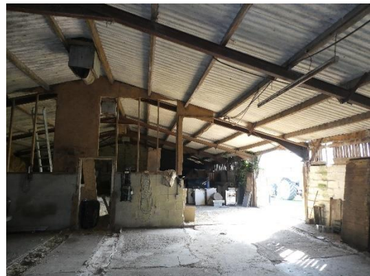
Photograph 4: Interior view of the shed
