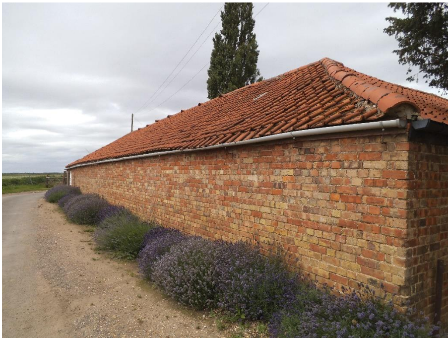
Barn 1 as seen from the road
