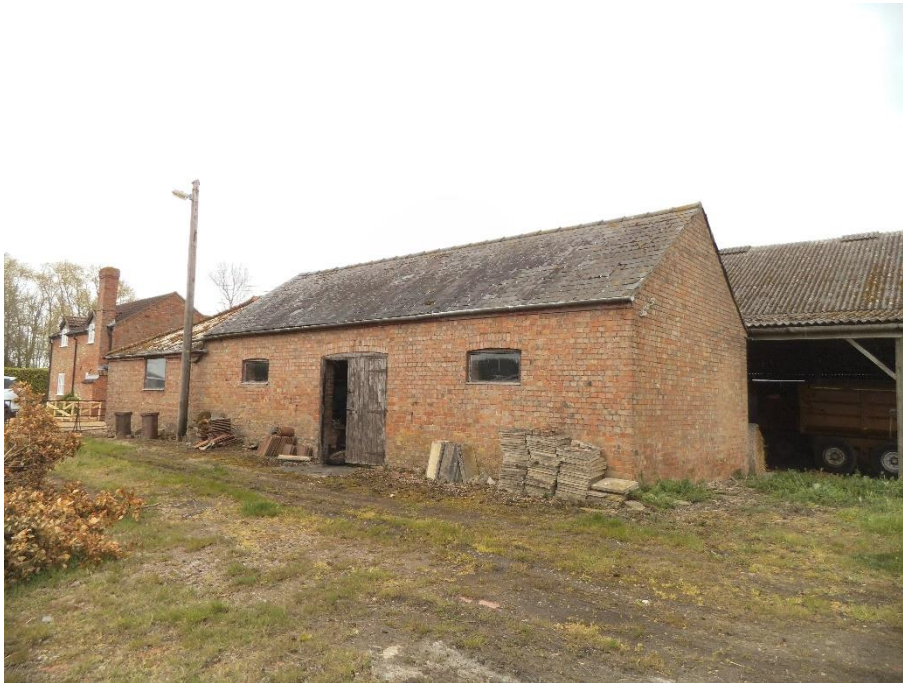
Barn 2 as seen from the rear.
