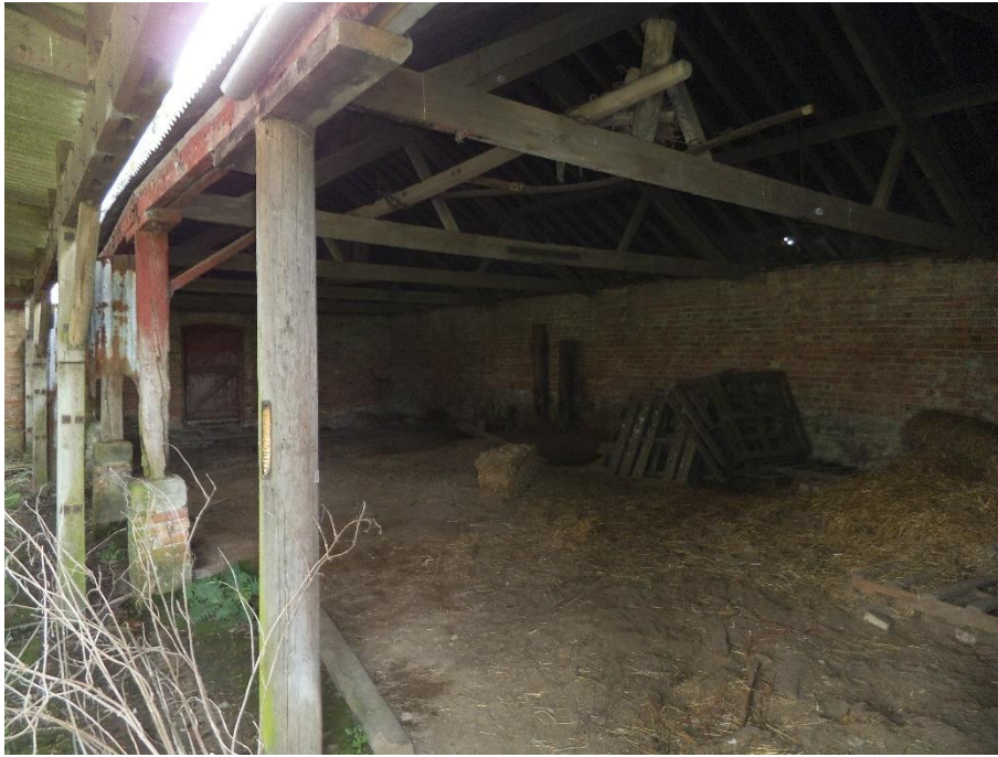
Barn 1 as seen from the rear
