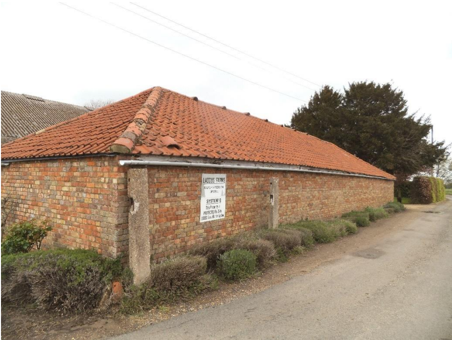
Barn 1 to be converted
