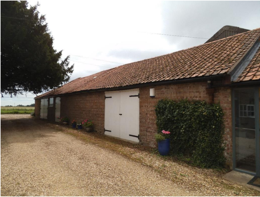
Barn 1 section to be converted to an annexe as seen from clients drive
