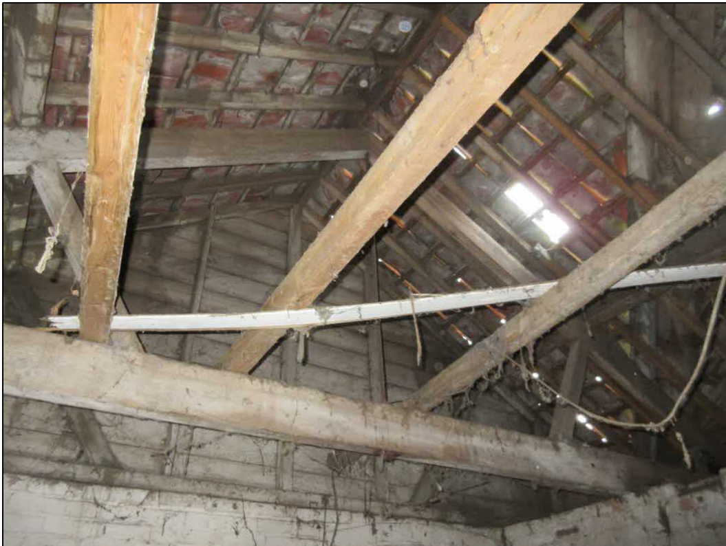
Photo 16. Unlined roof of barn 4
