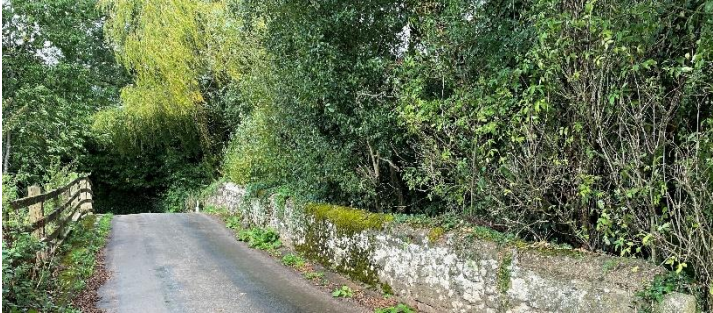
photo (left), looking west, over the bridge (02) towards the Site
