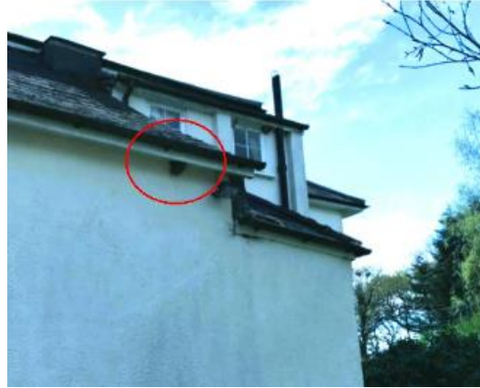
Plate 9. House Martin nest on northern elevation
