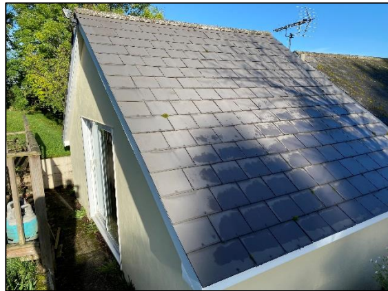
Plate 4: Area to be demolished (facing north-west)
