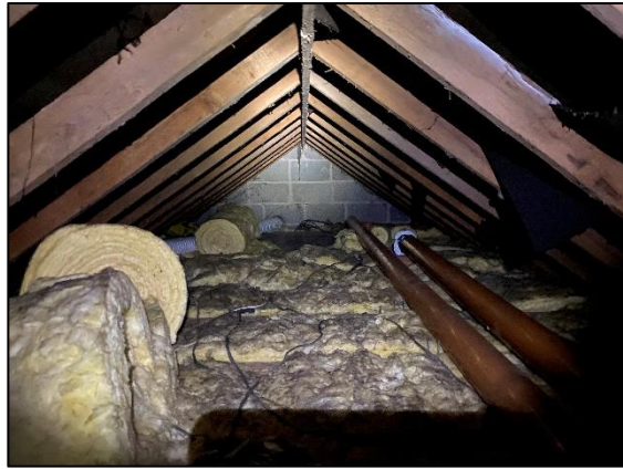
Plate 2: View of roof void over bedroom area
