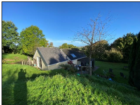
Plate 6: View of annexe (facing north-west)
