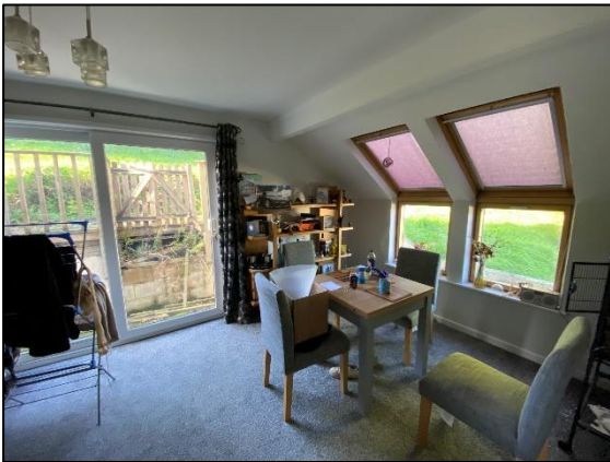
Plate 3: Area to be demolished
