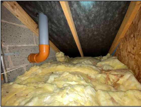
Plate 1: View of roof void over hall
