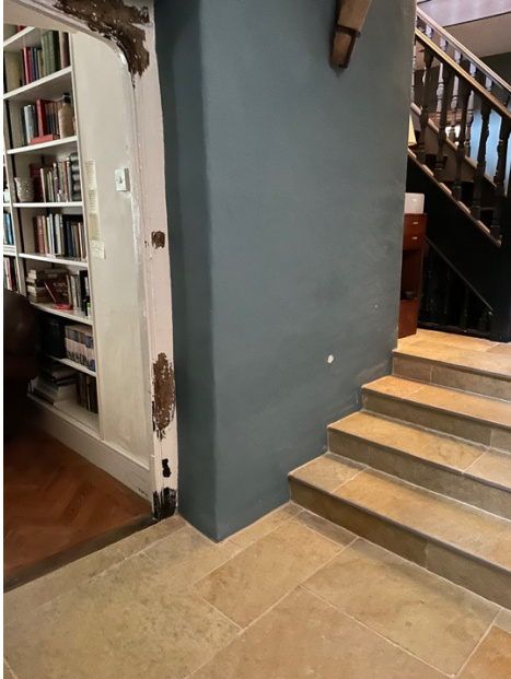
Photo 3.2. Door to the Library (on the floorplan). Note some paint removal to the door – with bottom of door frame having been recently replaced, and the new stone floor.
