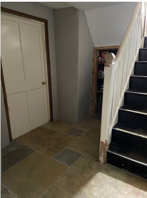
Photo 3.5. Door to Kitchen and back staircase. Note the door frames stripped of white gloss and the new stone tiles.
