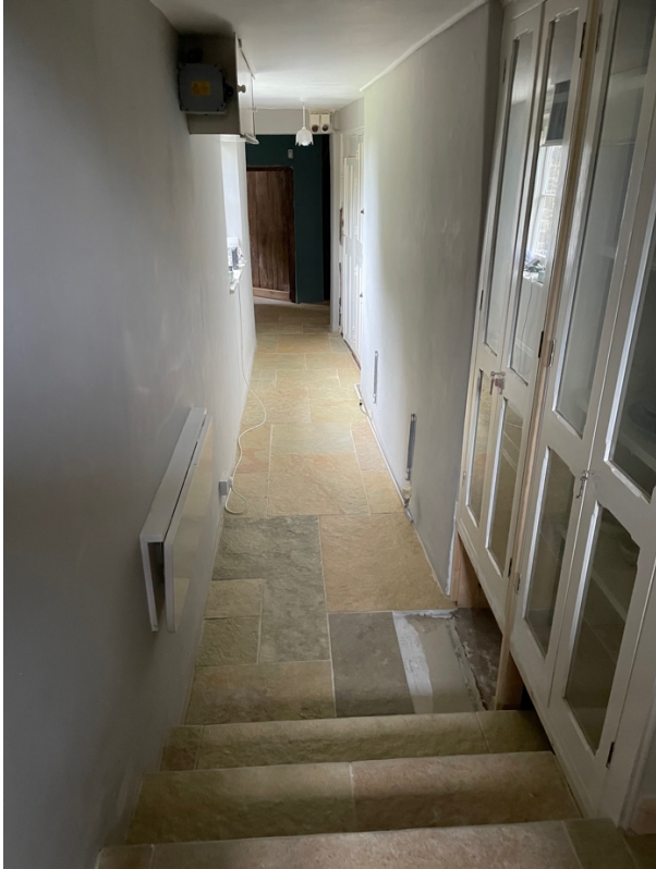
Photo 3.6. Back corridor. Note bathroom door stripped and the new stone tiles.
