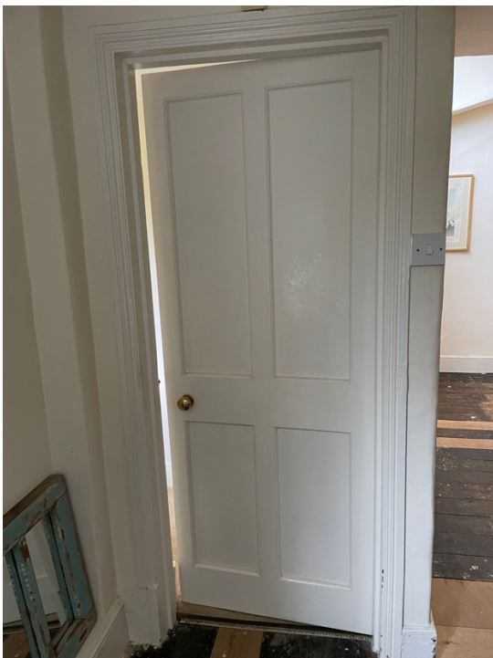
Photo 3.9. Door to WC to landing – plywood panel
