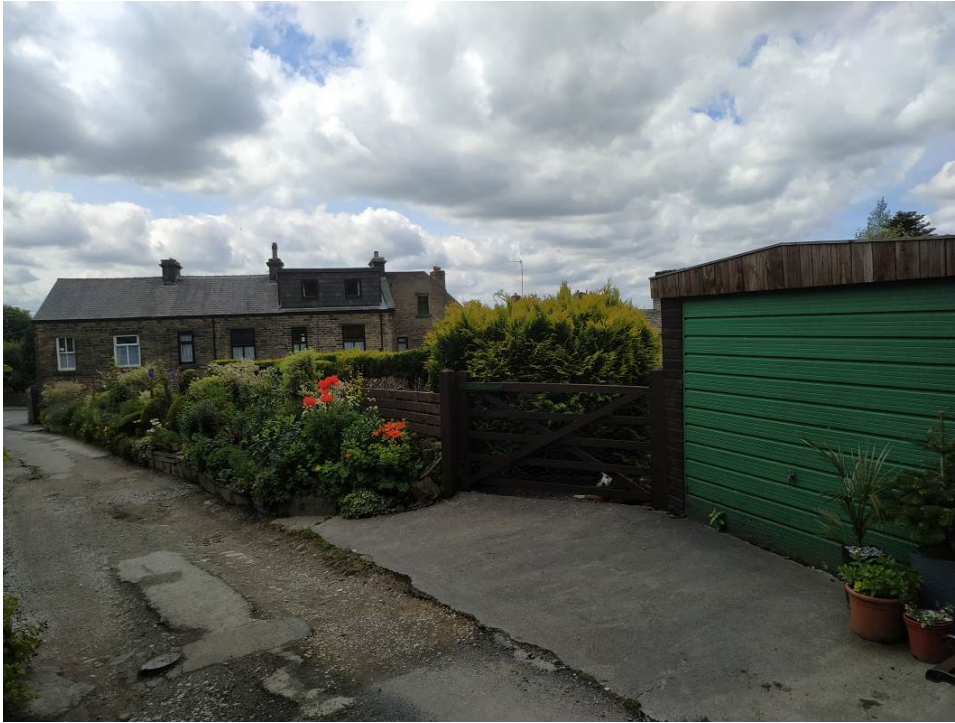
P2 Wainsgate Lane, looking south at backs of No.s 1 to 4 Ayre View and with subject site access and garage in foreground.
