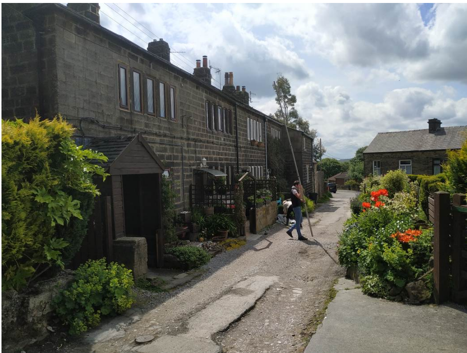
P3 Wainsgate Lane, looking south at fronts of No.s 1 to 5 Wainsgate Lane and with subject site access to the right of the foreground.
