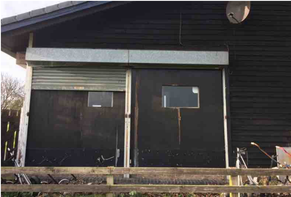
Figure 4 Existing Golf Pro Shop, side windows
