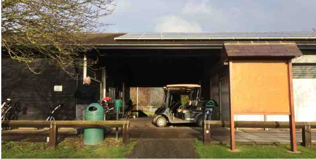
Figure 5 View of main entrance walkway and buggy parking
