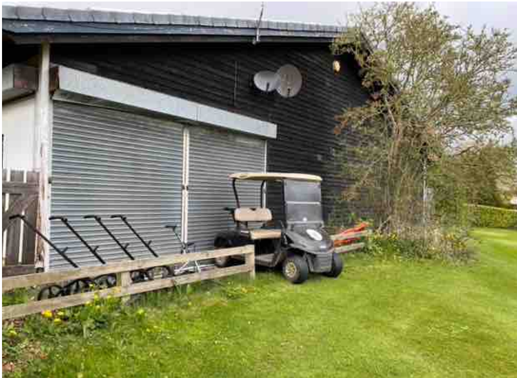
Figure 6 Pro Shop existing gable view
