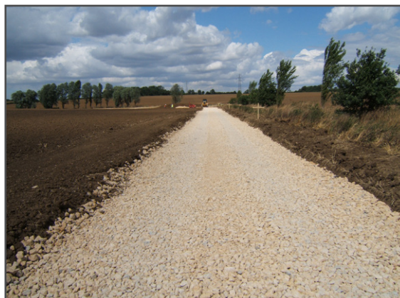
Plate 10 - Typical New Site Access Track
