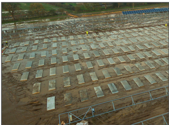
Plate 6 - Typical Surface Mounted 'Feet'
