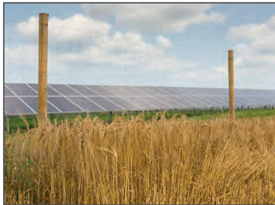
Plate 5 - Typical Security Fence
