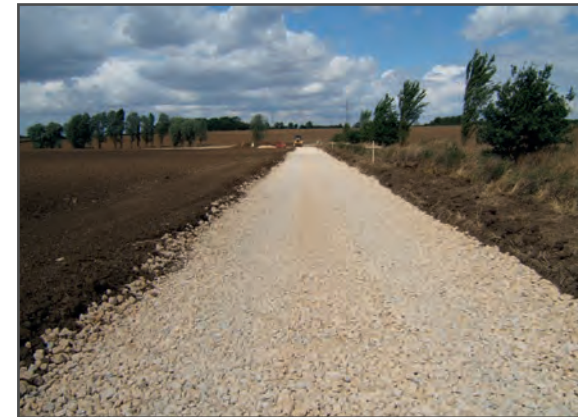
Plate 10 - Typical New Site Access Track
