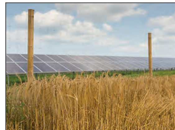
Plate 13 - Typical Security Fence
