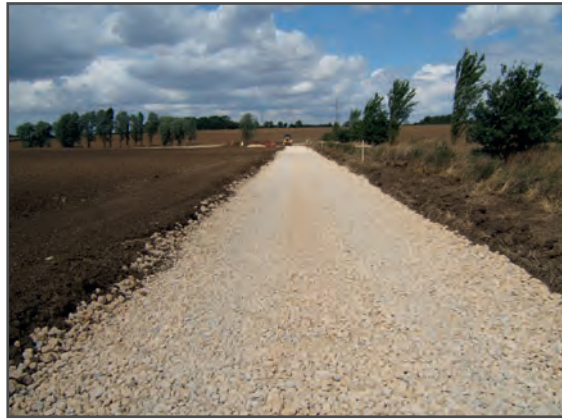
Plate 2 - Typical New Site Access Track
