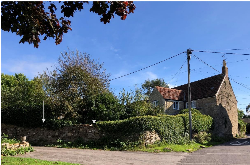
Fig.07 View of stone boundary wall with signs of previous opening indicated
