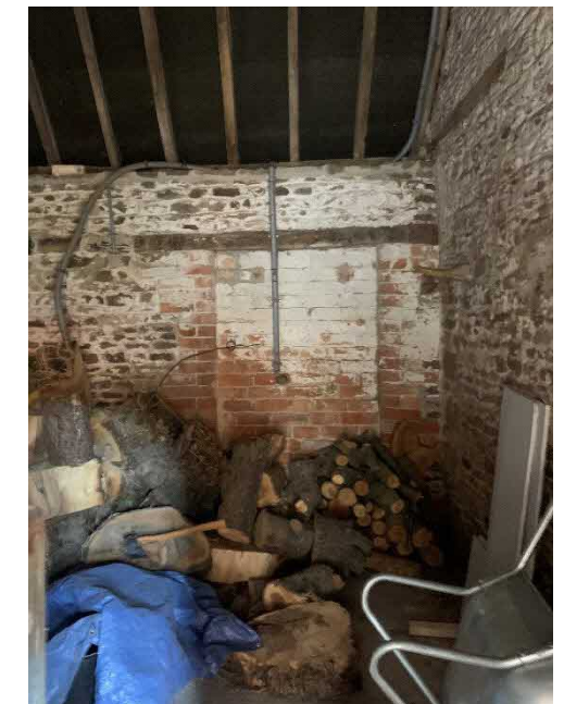
Photo 27: Photograph of existing condition of the stables
