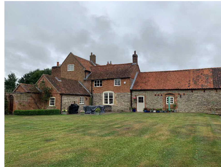
Photo 11: Eastern Elevation from the garden
