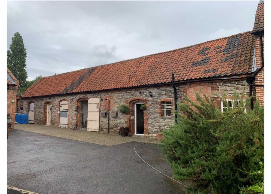
Photo 4: Western Elevation from the courtyard
