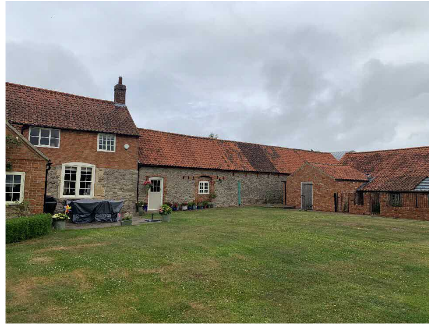
Photo 8: Eastern Elevation from the garden
