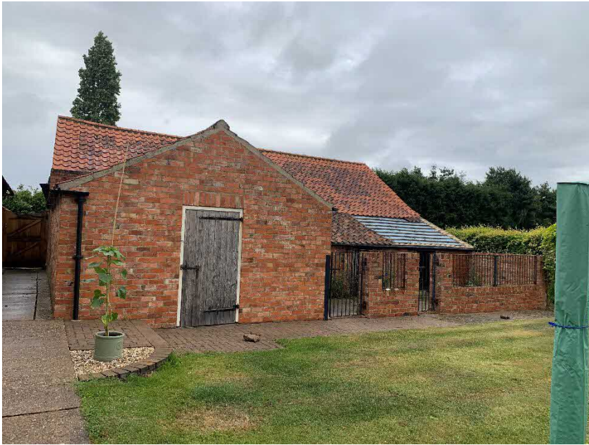
Photo 7: Southern Elevation of Kennels and Shed
