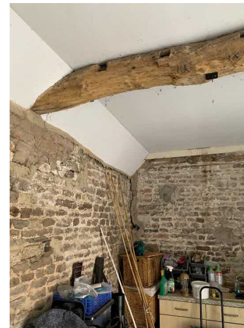
Photo 26: Photograph of existing condition of the stables
