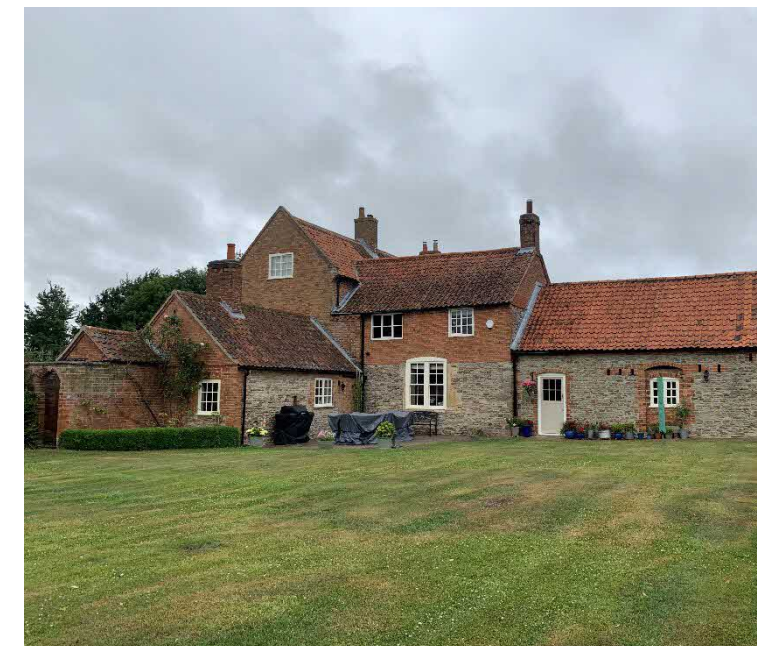
Photo 16: Phasing of buildings shown through material changes
