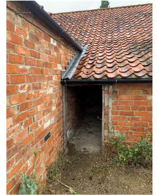
Photo 23: Evidence of condition of existing Cart Shed from the Piggery
