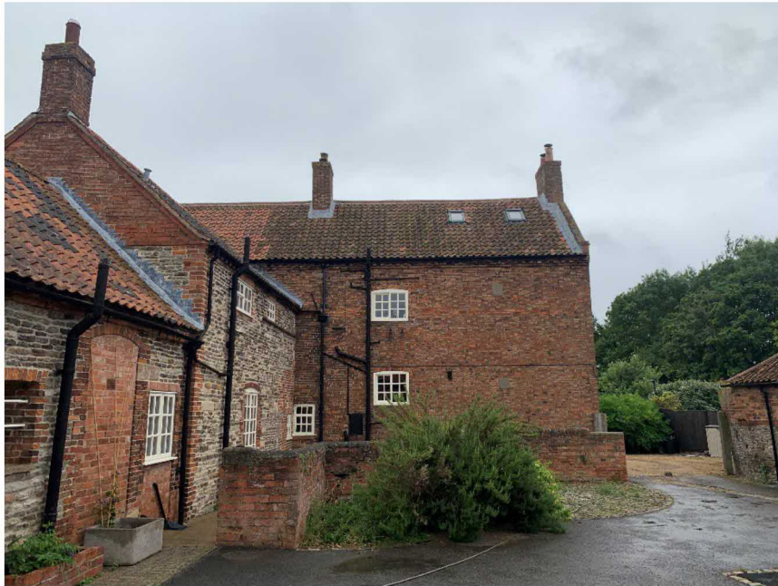
Photo 5: Northern Elevation from the courtyard Evidence of historically demolished shelter shed
