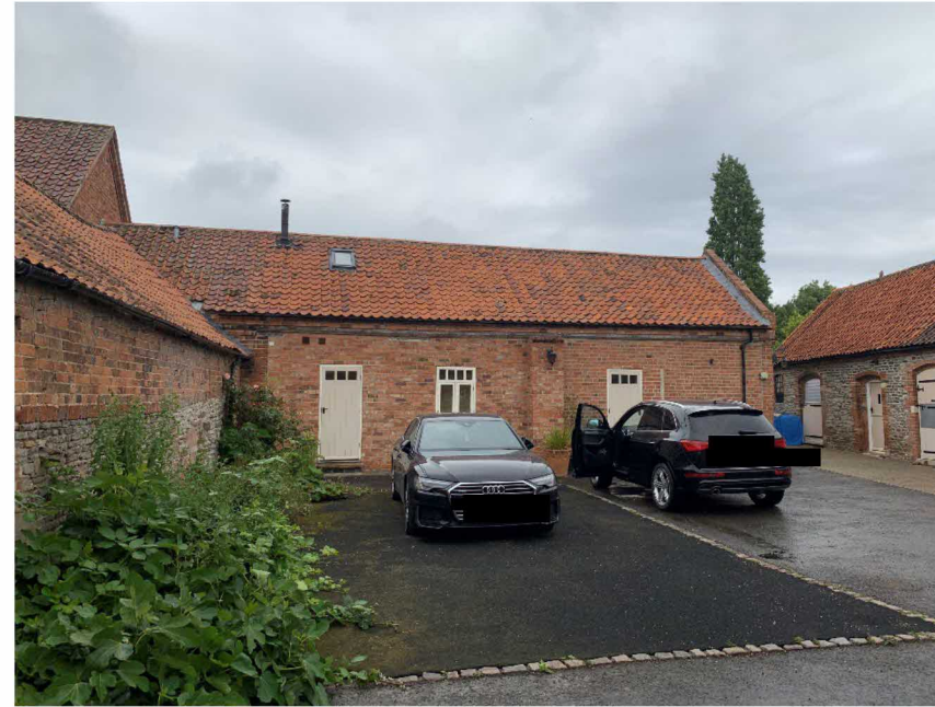
Photo 3: Southern Elevation of Barn
