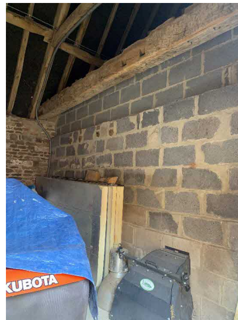
Photo 25: Photograph of existing condition of the stables
