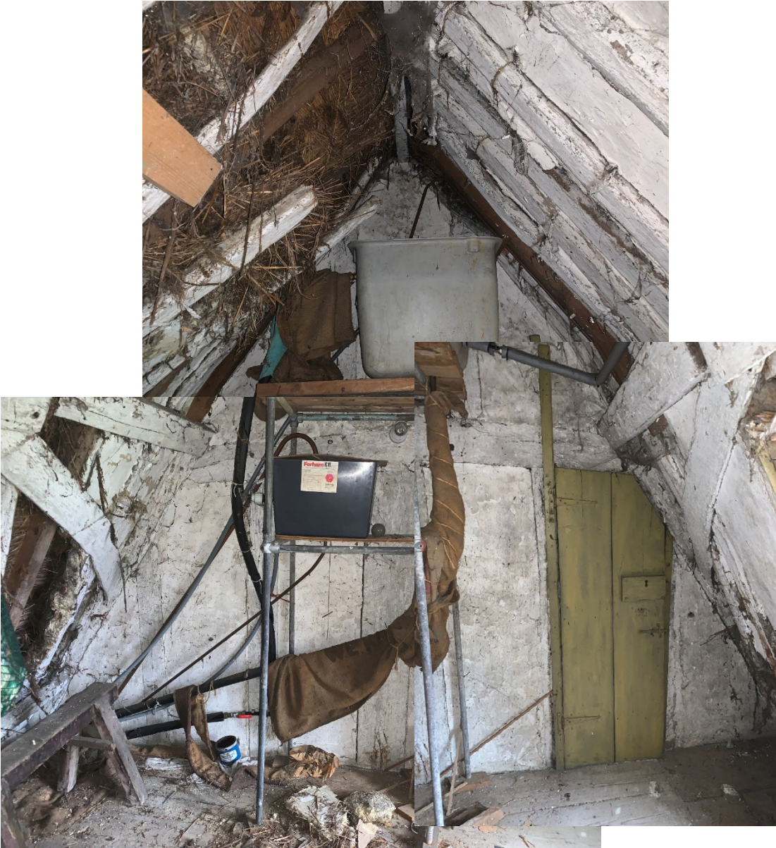
LOOKING TO CROSS WALL TOWARDS THE WEST
