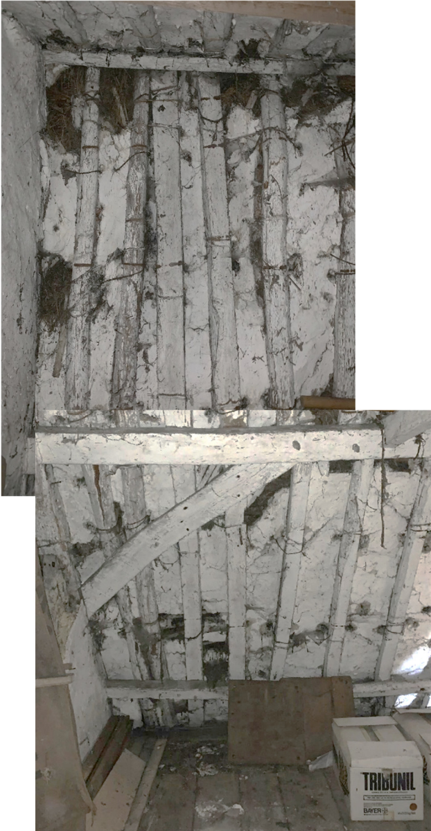
LOOKING TO SOUTH ROOF - LAST ACCESSIBLE BAY
