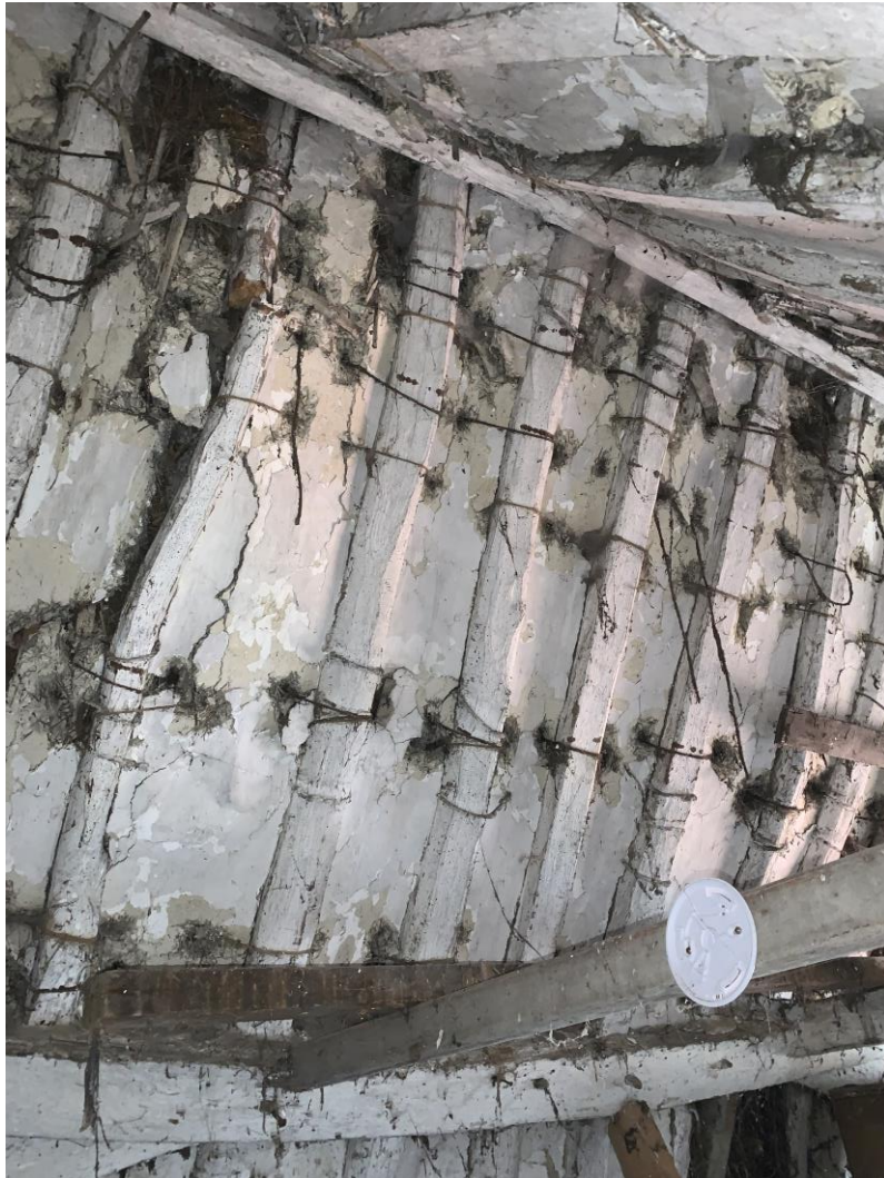
MODERN ROPE TIES AROUND PREVIOUSLY LIMEWASHED RAFTERS
