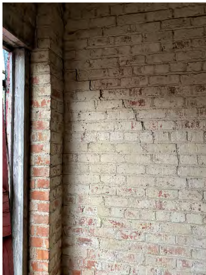
Movement towards West Elevation
