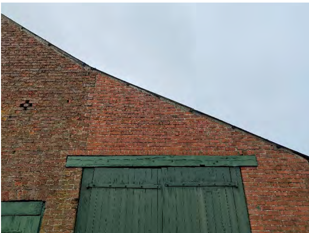
Movement in North Elevation
