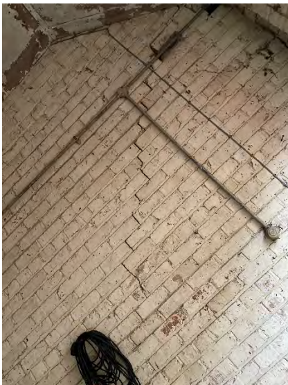
Movement towards West Elevation
