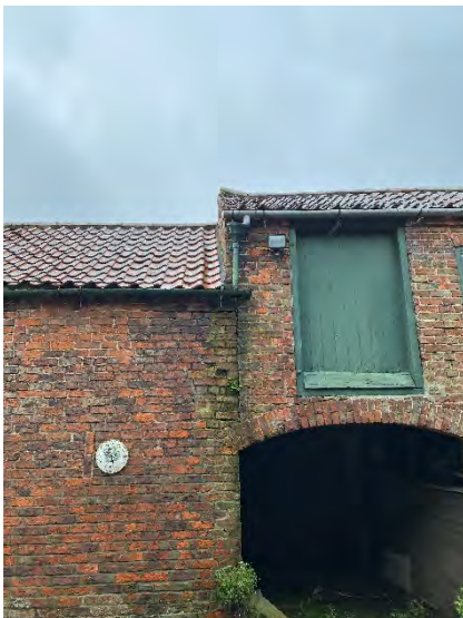
Arch bearing at junction of two storey section
