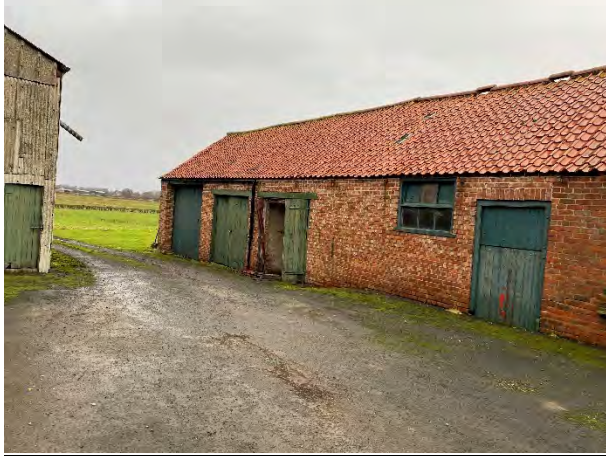
Courtyard view (West) shows undulating roof line
