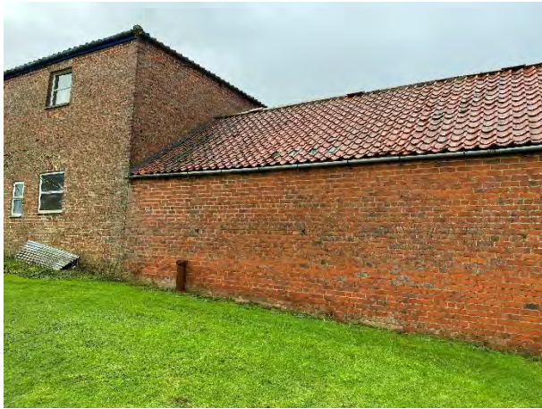
View of East Elevation
