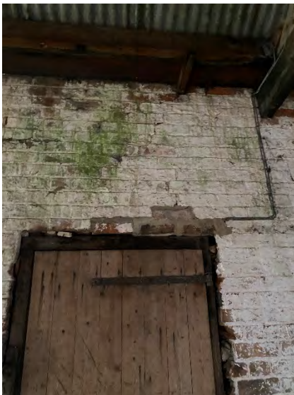
Covered yard Elevation with movement over lintel
