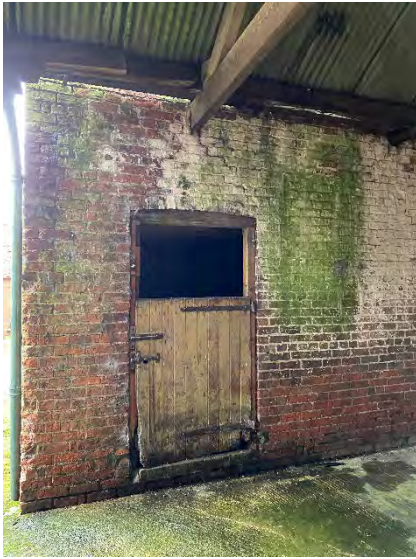
Covered yard Elevation with movement over lintel
