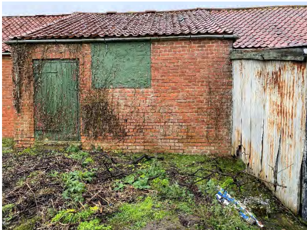
View of East Elevation
