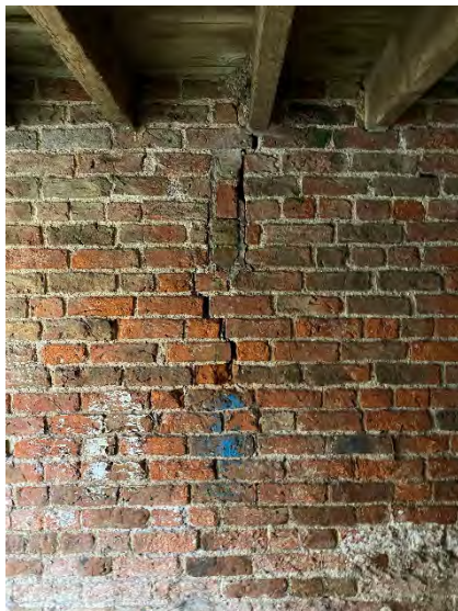
Vertical crack
