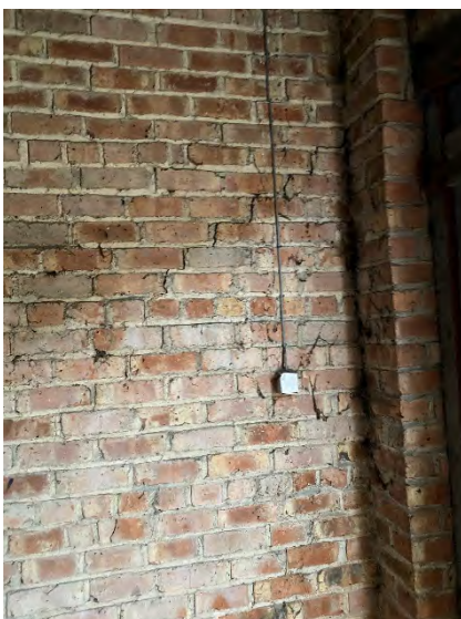
Movement towards West Elevation
