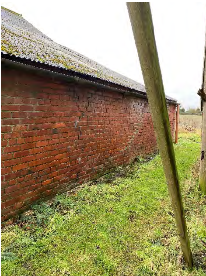
Movement in North Elevation
