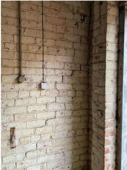
Movement towards West Elevation
