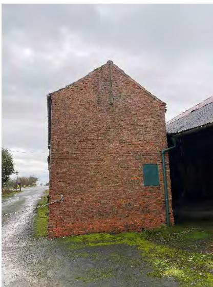
View on North Gable
