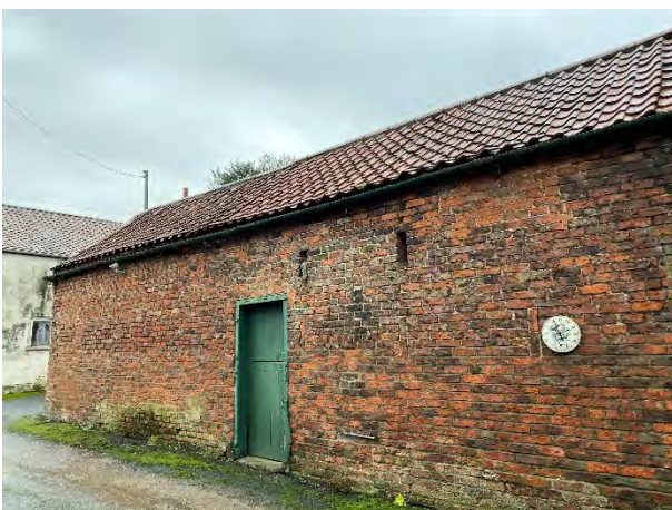
View on courtyard eaves wall
