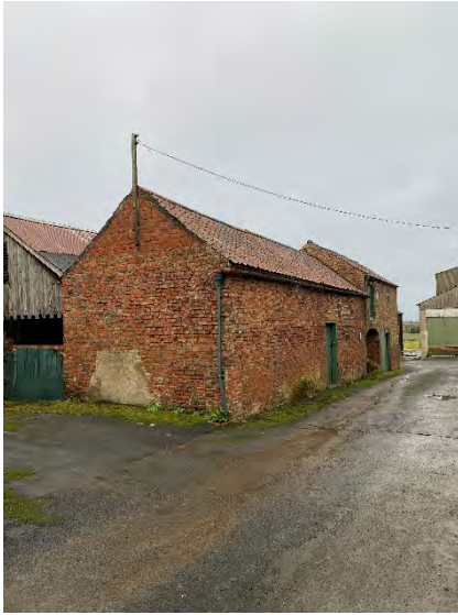
View from Courtyard
