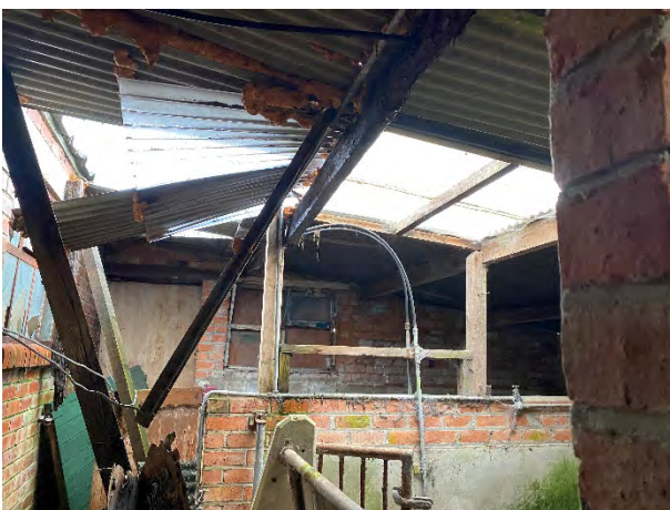
Roof missing/failed
