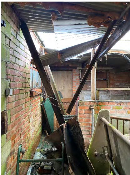
Roof missing/failed
