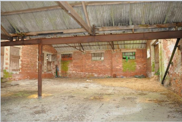
Plate 39: View to Building H across covered yard
