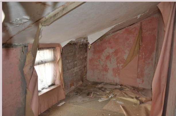
Plate 26: Example of size and room volume of rear first floor bedroom
