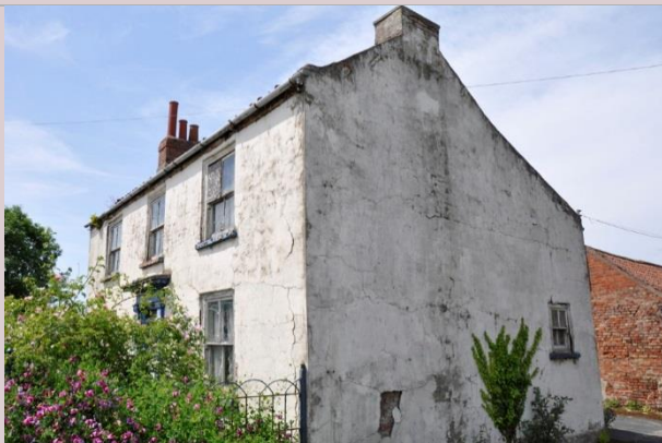
Plate 21: Gable elevation illustrating roof slope to rear
