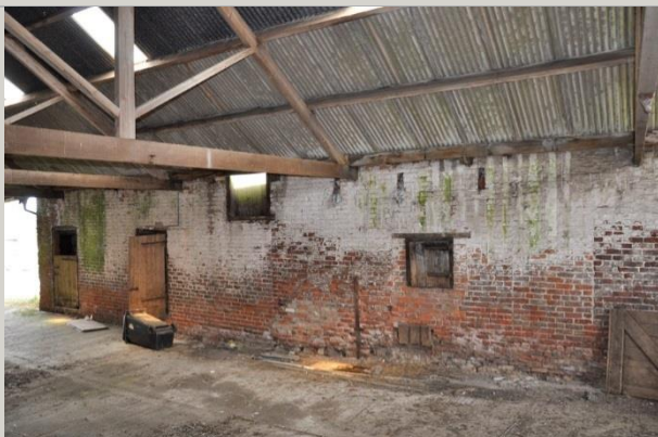
Plate 14: Elevation facing covered yard shows a building break between the two and single storey components but also within the single storey range suggesting phases of rebuilding with various stable doors linking the historical farmyard to this range
