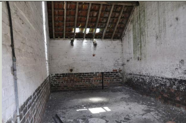
Plate 8: Example of a loose box
