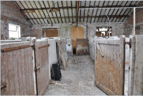
Plate 3: Internal view with eight pig stalls formed from concrete blockwork with timber doors
