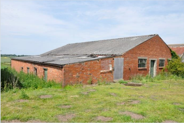
Plate 37: South elevation shows that it is later addition to the piggery to the left of this image
