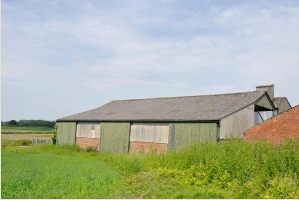
Plate 43: Cattle shed is a mixture of brickwork and corrugated sheeting with sheet roofing
