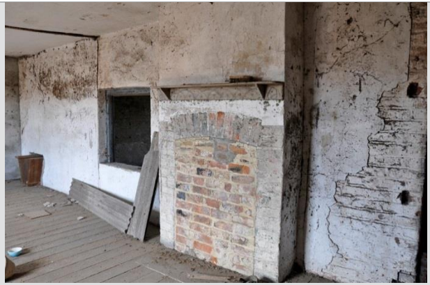
Plate 34: Blocked fireplace at first floor above open fronted ground floor bays
