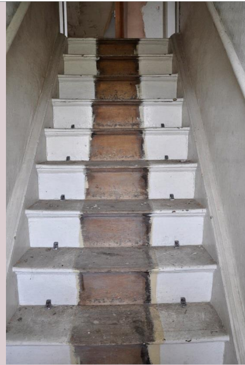
Plate 23: Primary straight flight timber stair at front
