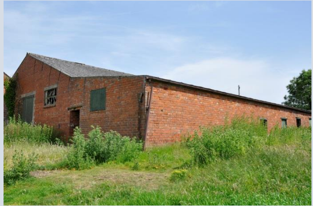
Plate 38: The design of Building H is more utilitarian than the adjacent piggery with simpler appearance to openings
