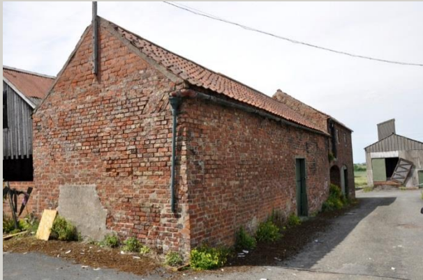
Plate 12: Single storey range with rebuilt roof and evidence of tumbled brickwork suggesting the current south end is the original south gable
