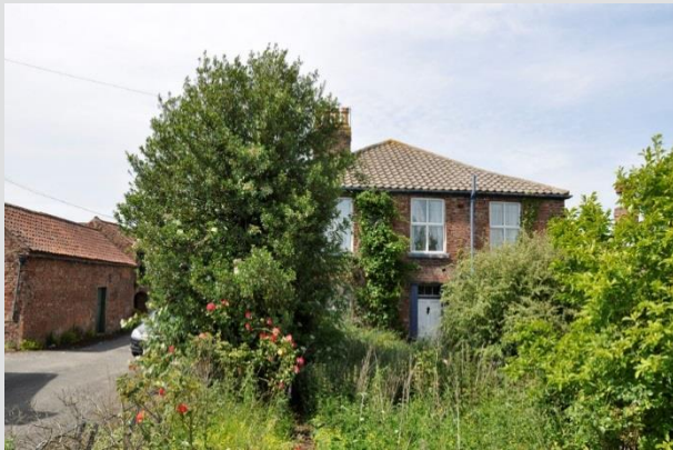
Plate 27: Front elevation viewed across overgrown front garden with decorative metal railings and three bay frontage with brick elevation, UPVC window units and hipped roof with later cover
