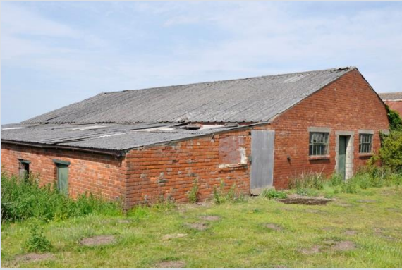
Plate 1: Piggery south elevation with adjoining Building H in foreground. Note use of decorative concrete to door opening and concrete lintels and brick sills to timber framed casement windows
