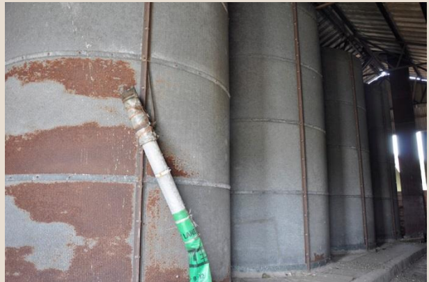
Plate 46: Silos within shed
