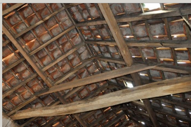
Plate 18: 20 th century roof structure to two storey range
