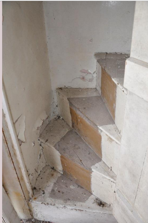
Plate 24: Secondary staircase with winder in timber enclosure to rear
