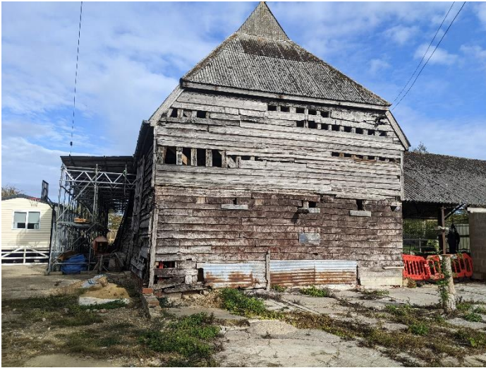
Photo 1 South gable of barn
