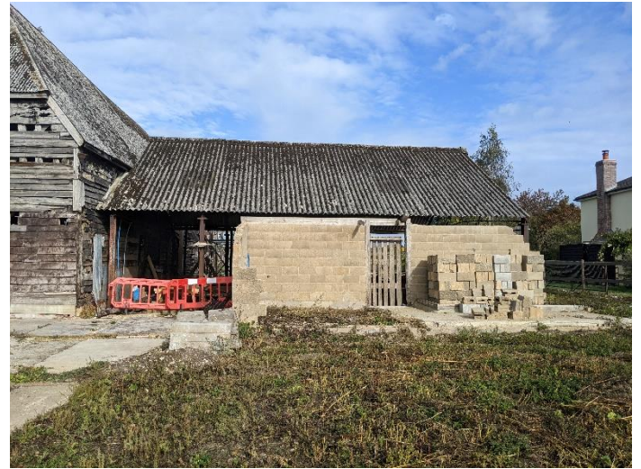
Photo 2 Side extension to the timber framed barn
