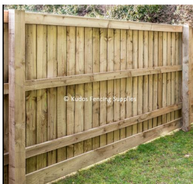
Vertical timber boarding onto frame on the inside face of the enclosure
