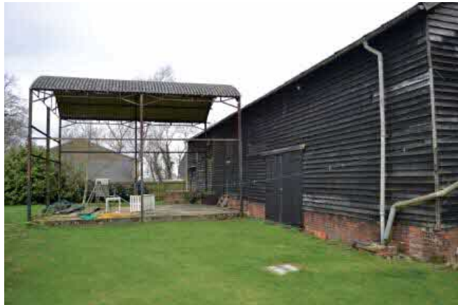
Dutch barn addition
