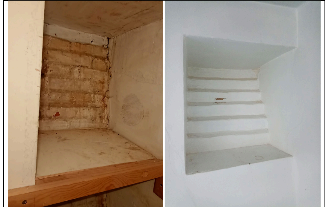
Stepped shoulders to flank walls of chimneys inside the en suite (to be retained).
