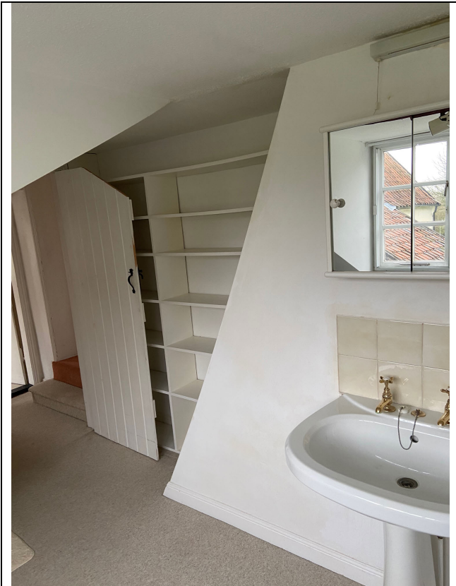
Sloped side of chimney above Aga chimney as it flues into main stack (to be retained).
