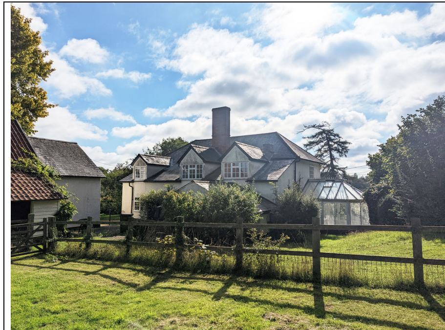
The two chimneys as viewed externally. Both stacks will be retained.
