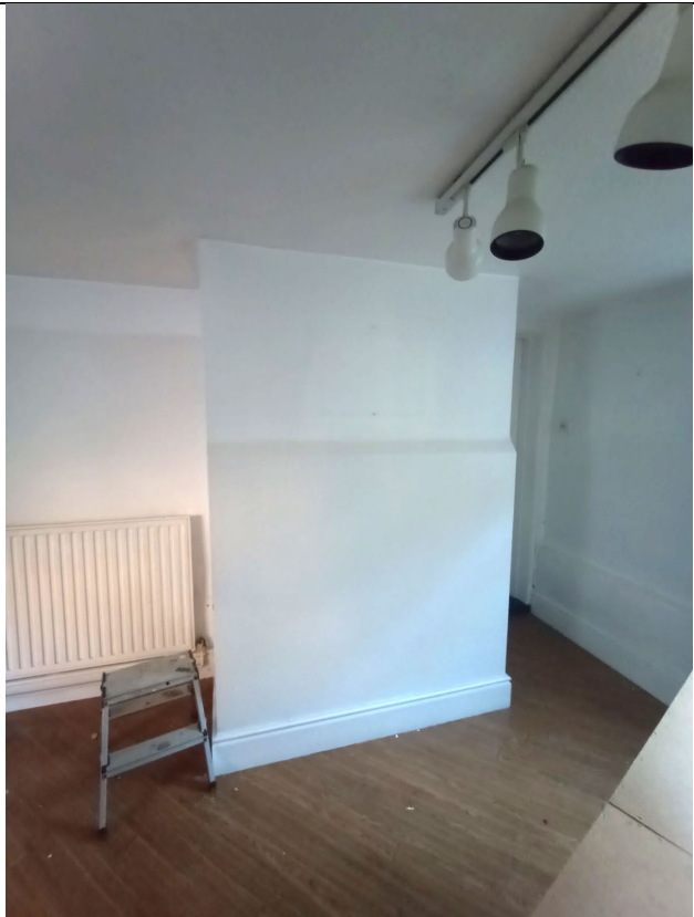
Rear of chimney proposed for removal in the present-day kitchen.
