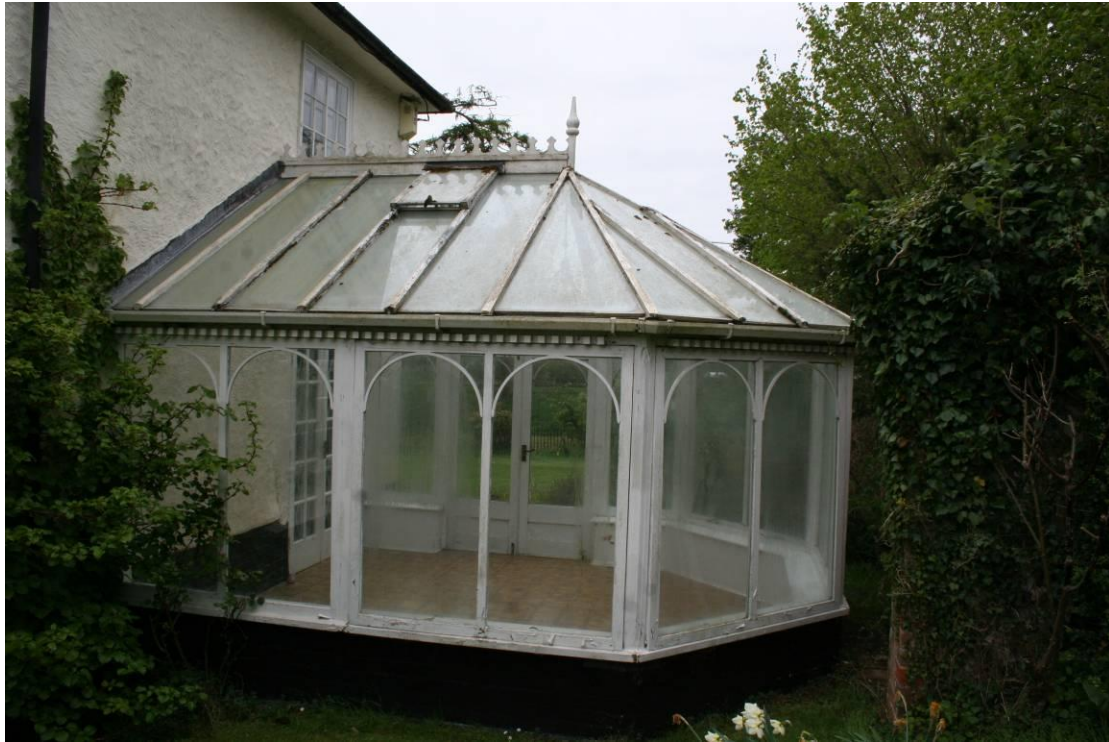
The north and west elevations of the conservatory.
