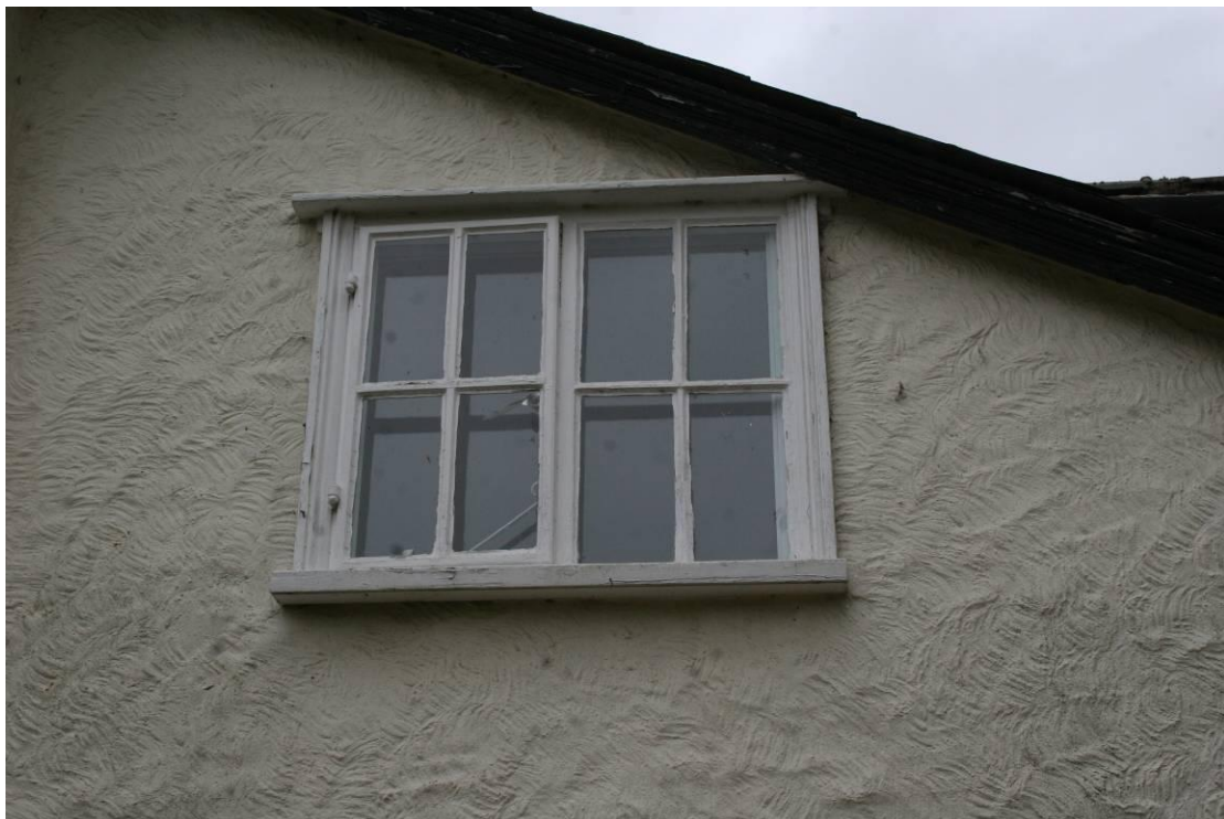
Upper floor window with metal frame.
