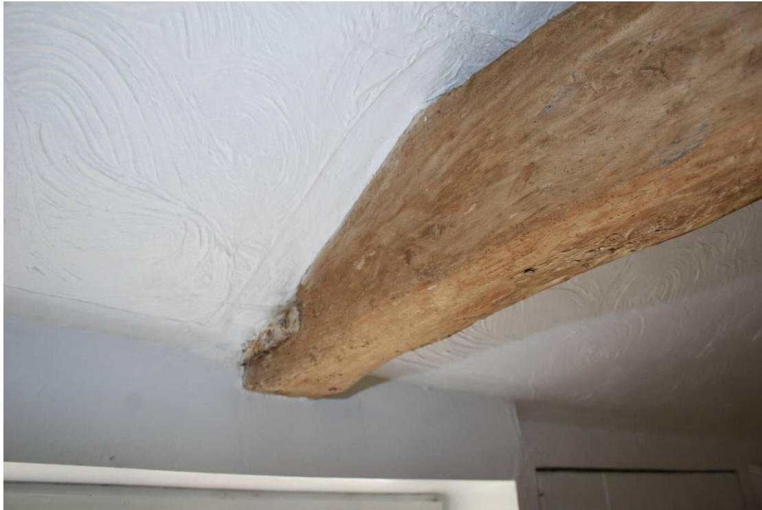
The eastern end of the tie-beam with short iron tie.
