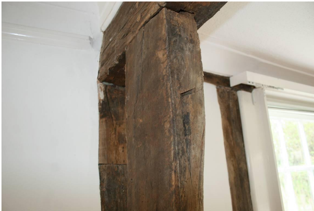
Stud with deeply cut wattling dart. Southern end of wall frame.
