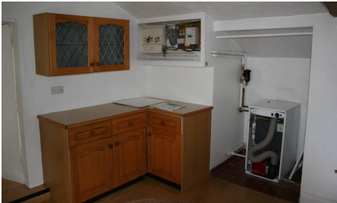
Looking SW in the Utility Room.
