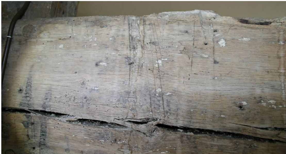
Taper burn marks and strike marks on the top-plate.
