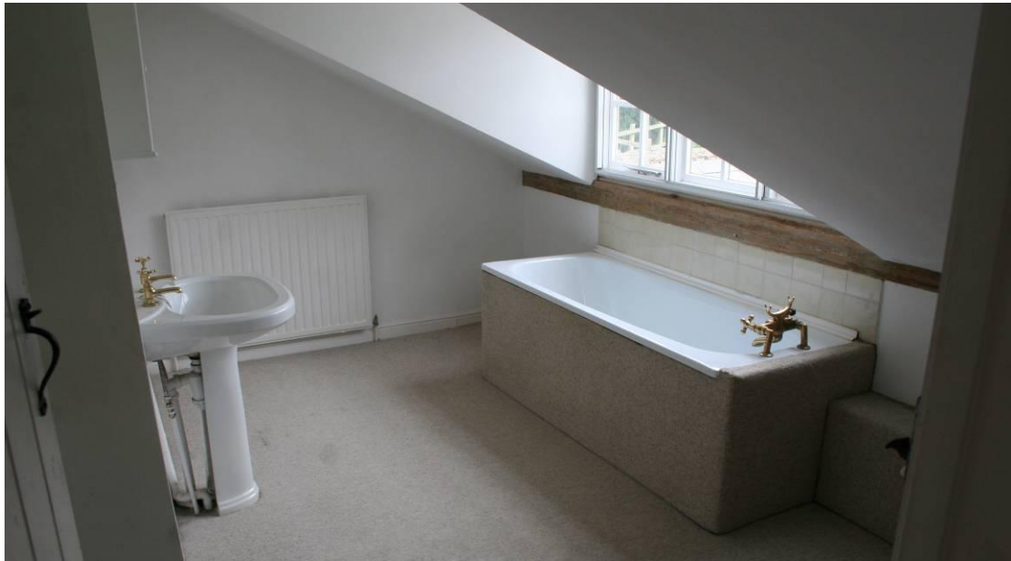
Looking W in Bathroom 2.
