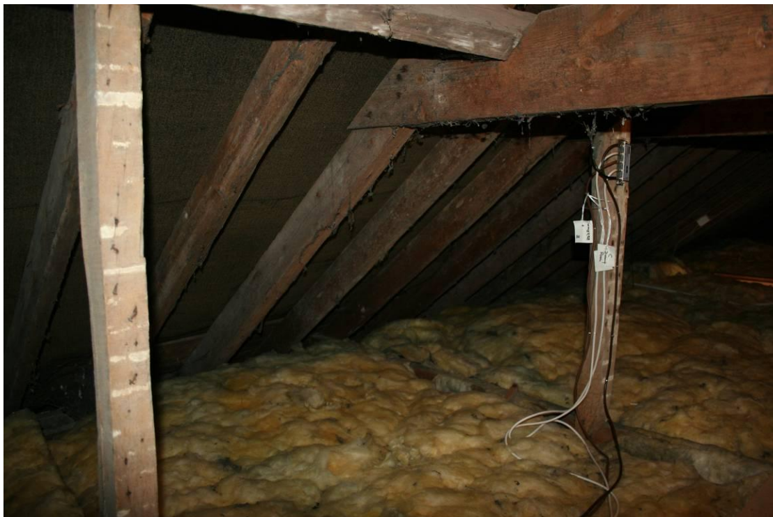
Reused studs used as hangers for the ceiling structure.
