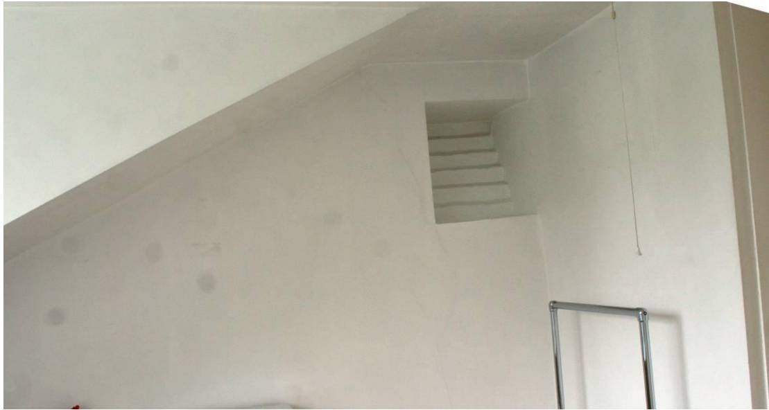
The east wall of the Bathroom.
