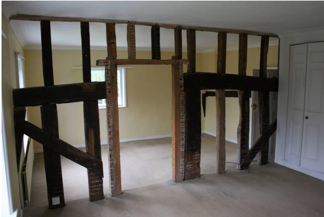
Looking W in Master Bedroom 1.
