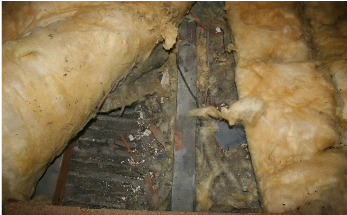
Machined softwood ceiling joists with lath and plaster.
