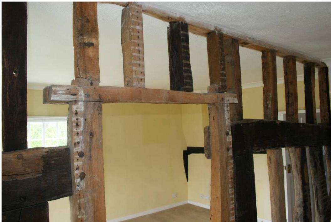
Detail of the inserted doorway in the top-plate.
