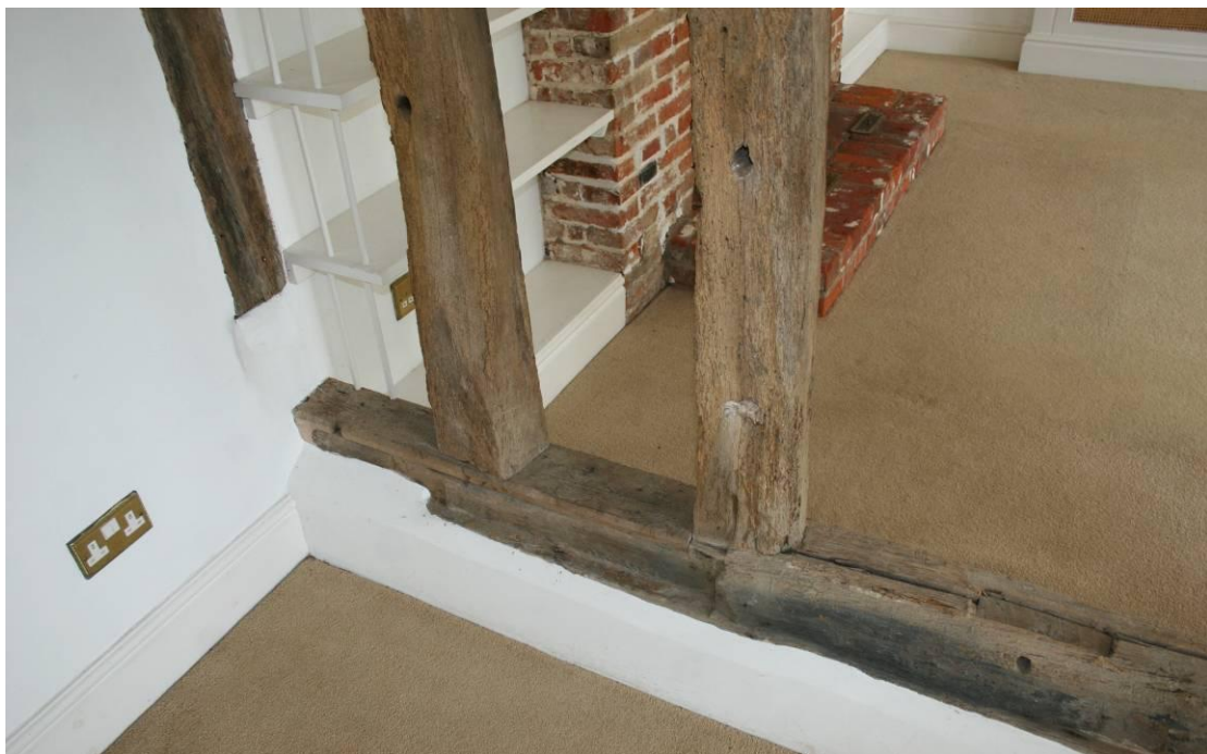
The soleplate is rebated for a doorway.
