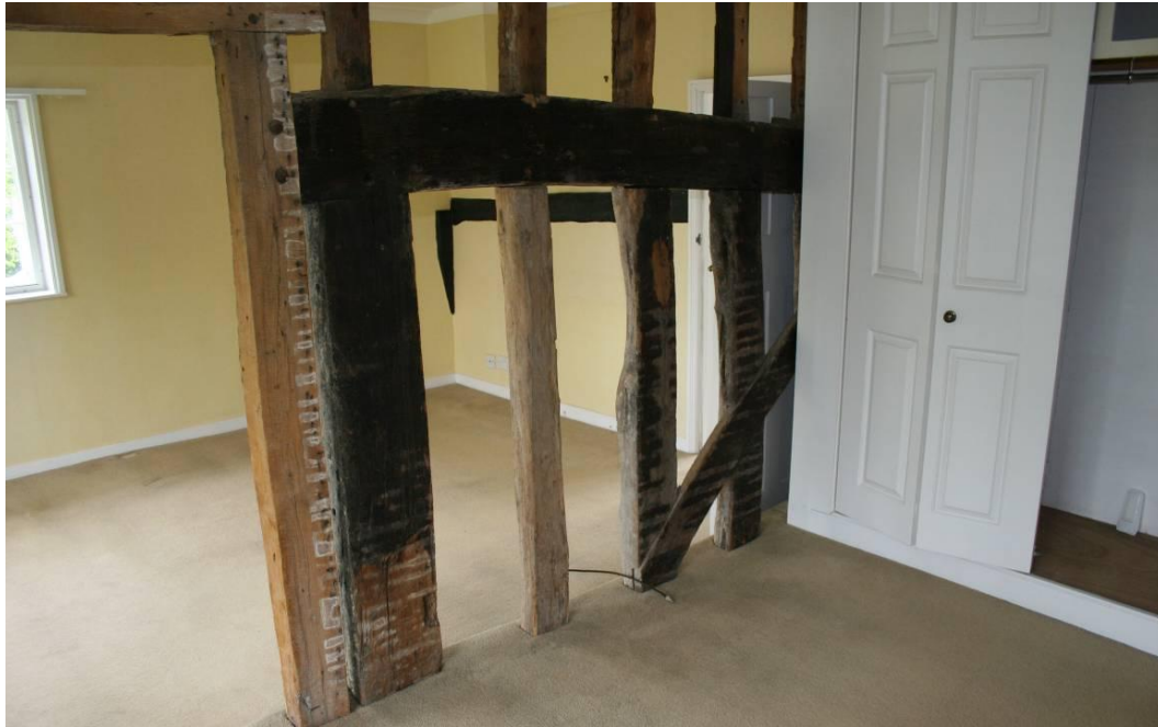
The light colour stud indicates an earlier opening. Looking W.
