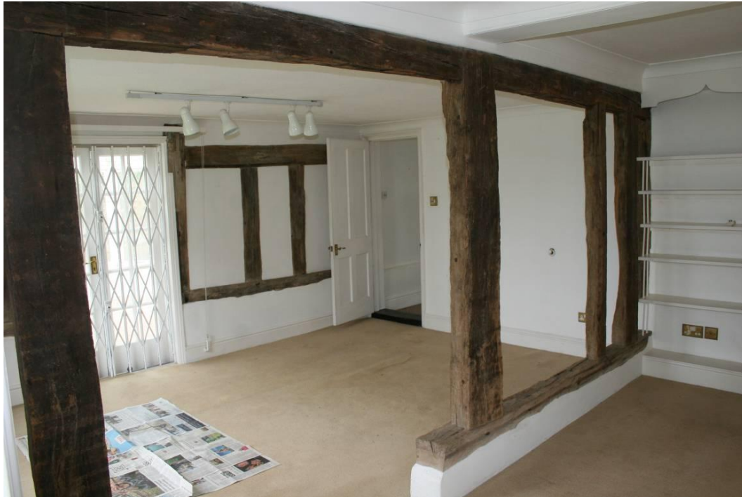
The dividing wall has been largely removed.
