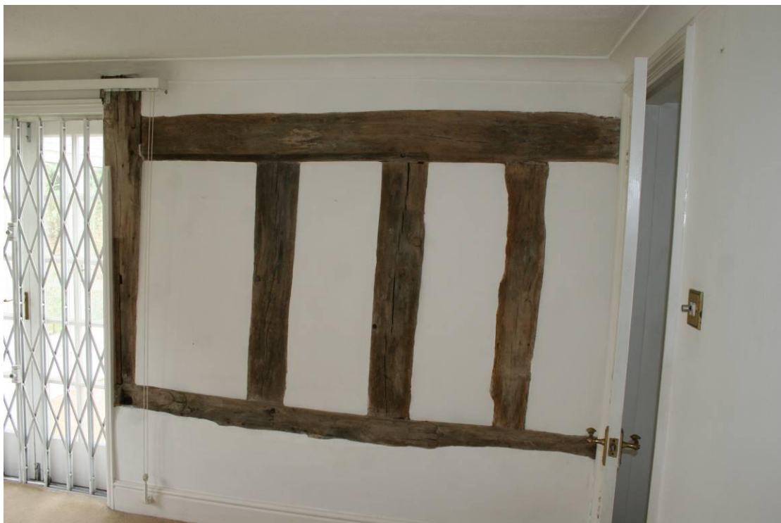
The external western wall frame.
