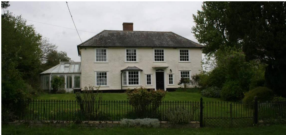
The south elevation of the House.
