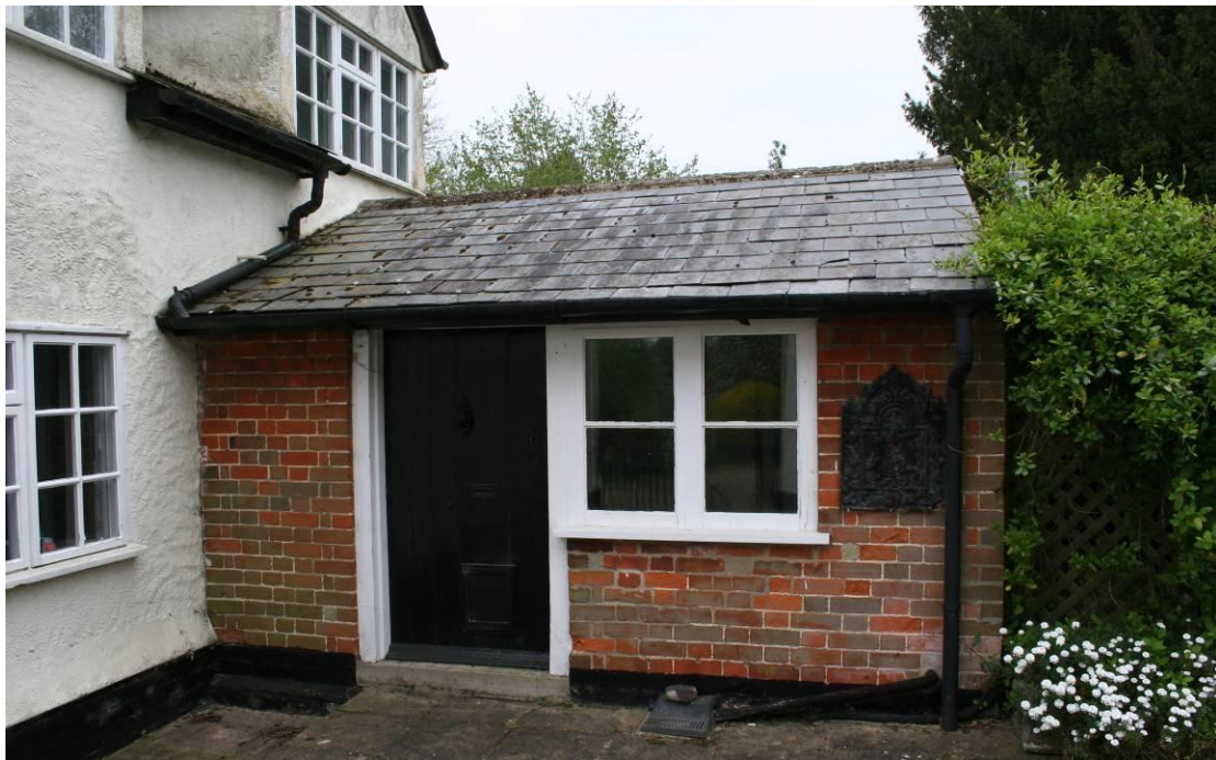
East elevation of the Outshot.
