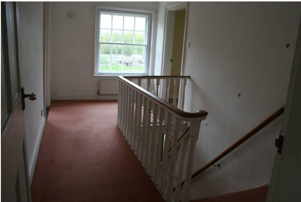
The first floor banister rail looking S.
