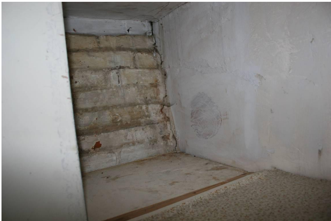
The flank of the western firestack.
