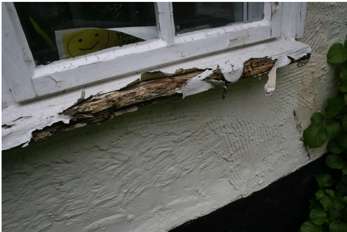
Low quality timber was used in the LC20th casements.
