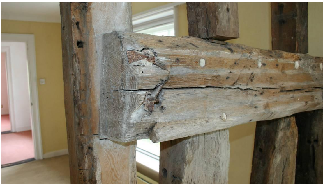
Detail of the forelock bolts.
