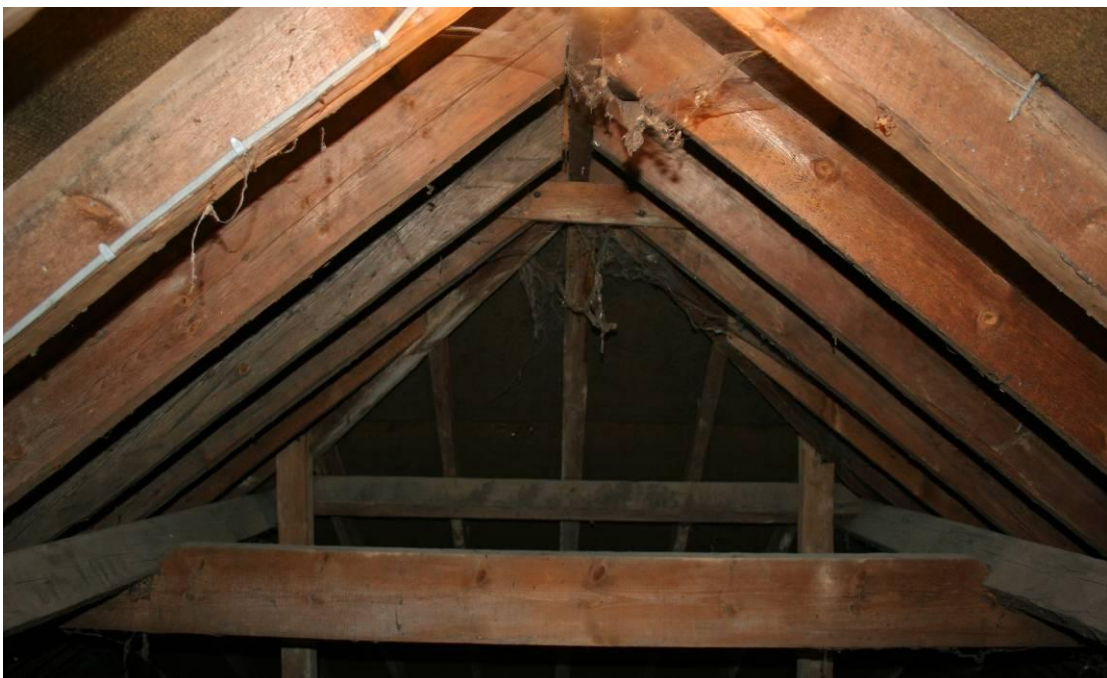
Looking W in the roofspace.
