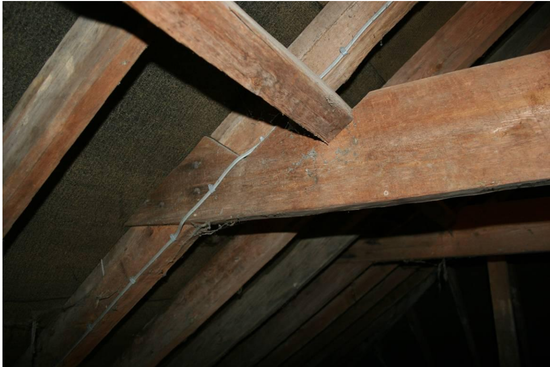
Detail of the collars and principal rafters.
