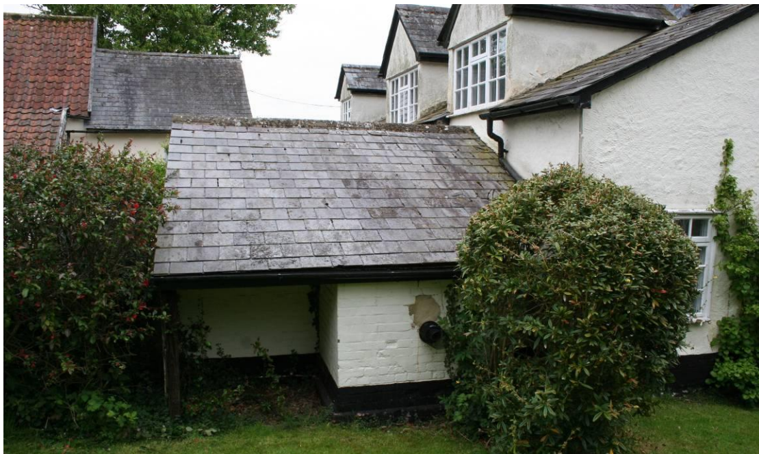
The west elevation of the Outshot.
