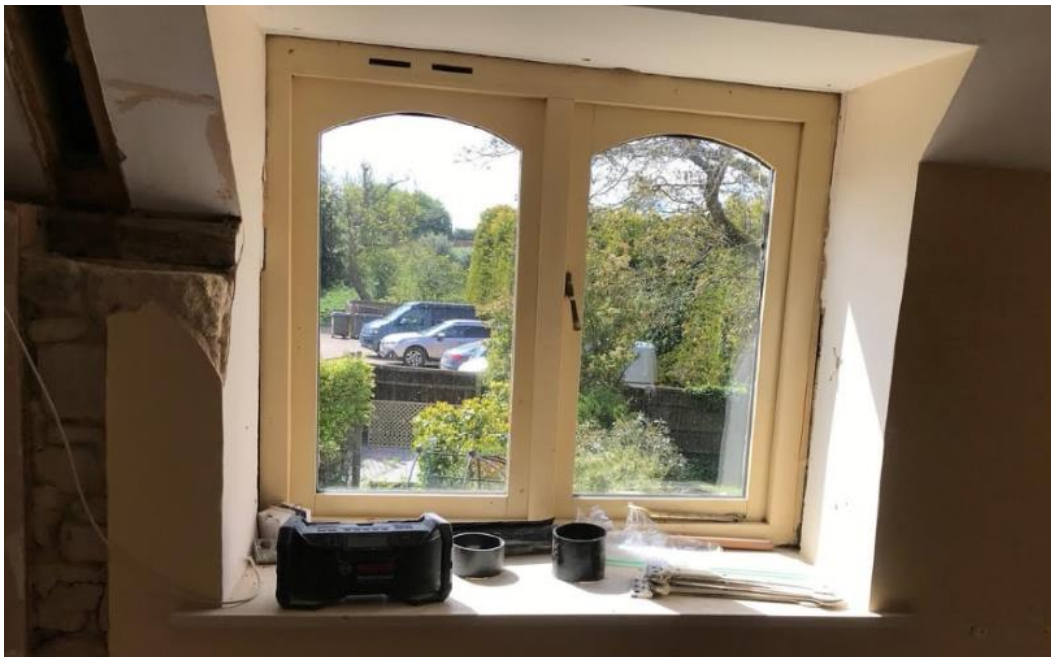
Pre-existing first floor double glazed timber window
