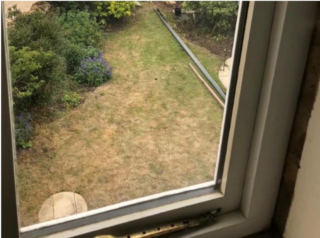
Two panes of glass of pre-existing fitments are clearly visible
