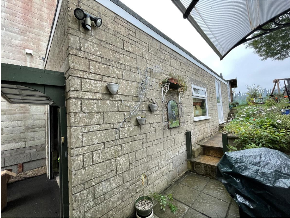
Fig. 4 –Side elevation of existing garage
