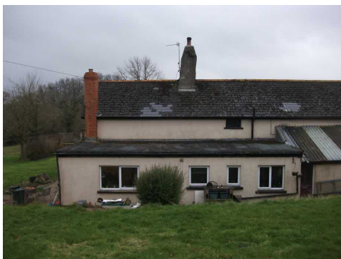
Existing Rear Flat Roof & Corrugated Iron Roof.
