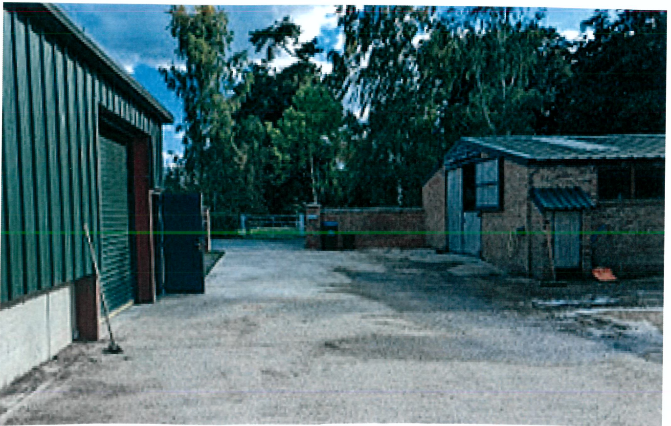
VIEW FROM NORTH THE BUILDING ON THE LEFT IS TO BECOME A GARAGE FOR THE RESIDENTIAL CONVERSION OF THE BUILDING TO THE RIGHT
