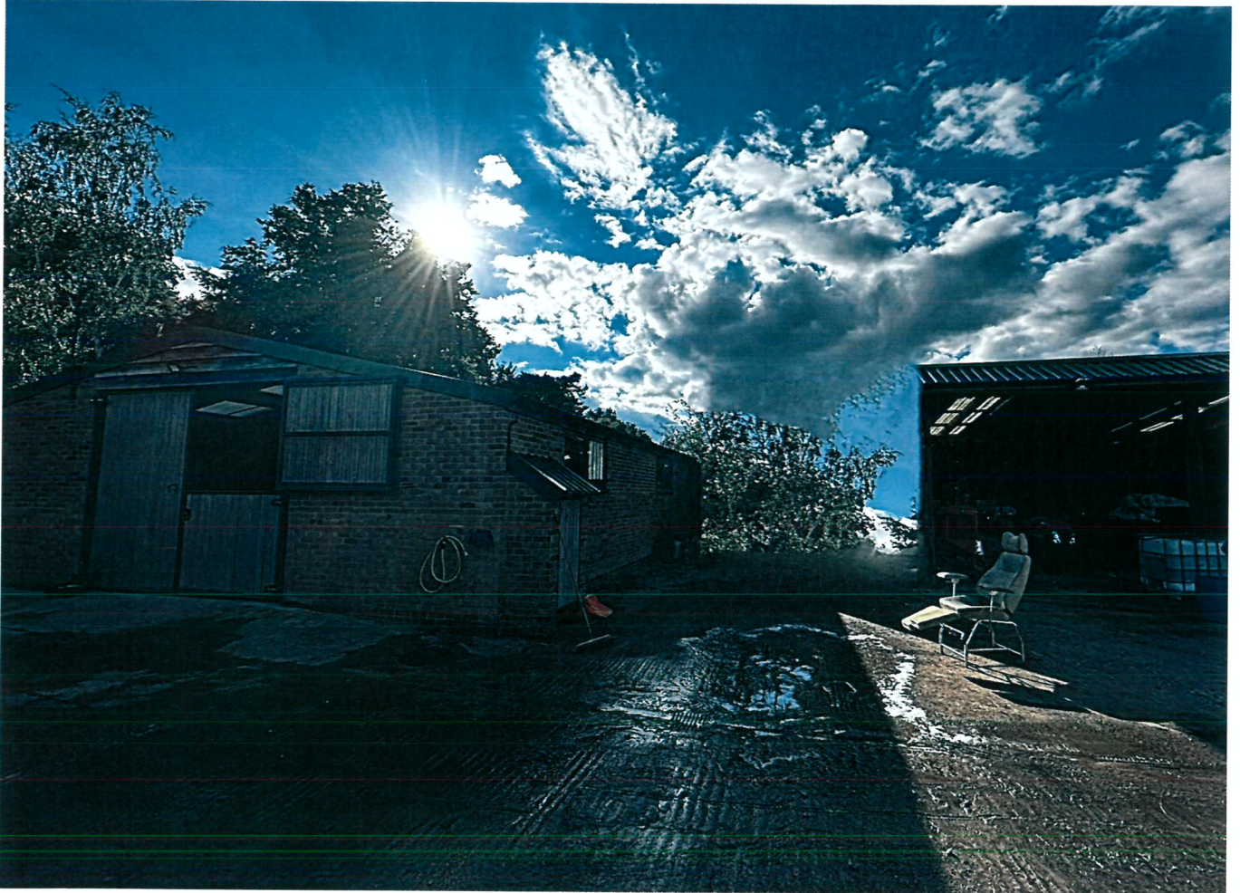
EDITED PHOTO SHOWING GAP BETWEEN RESIDENTIAL CONVERSION AND STORAGE BUILDING FOLLOWING DEMOLITION OF ONE BAY OF THE EXISTING OPENFRONTED STORAGE BUILDING
