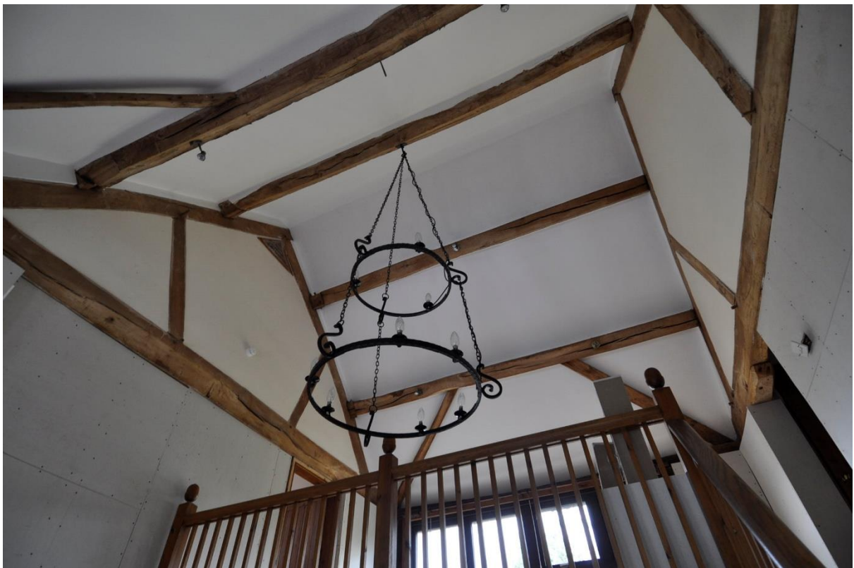
Ceiling above galleried landing, looking south
