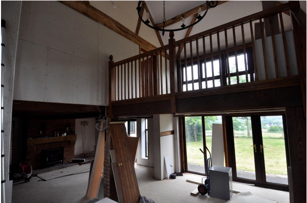
Galleried landing from living room, looking south
