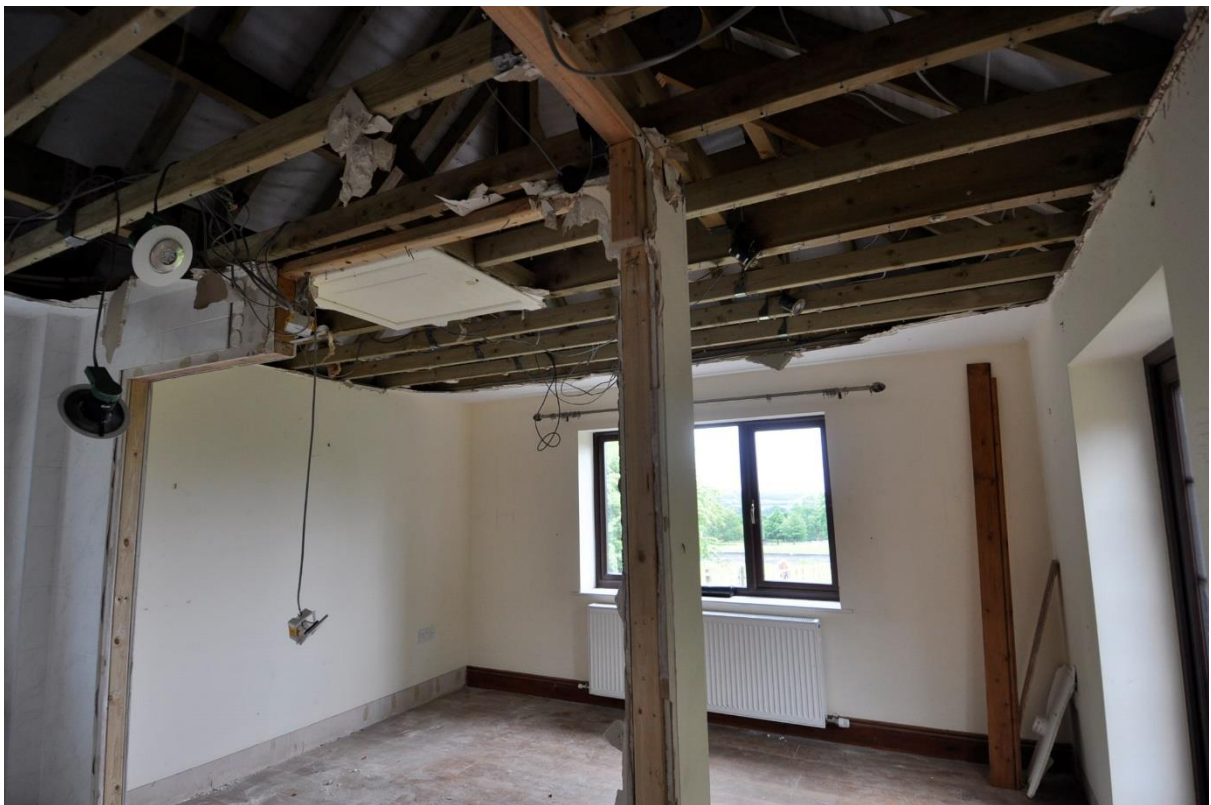
Annexe living room looking south
