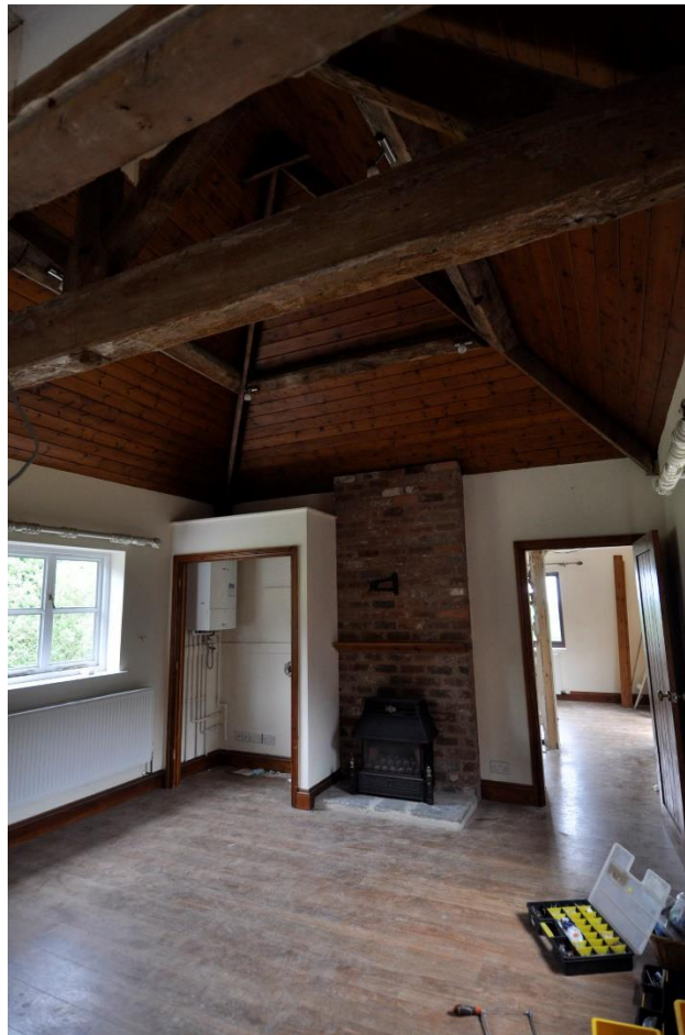
Annexe living room looking south
