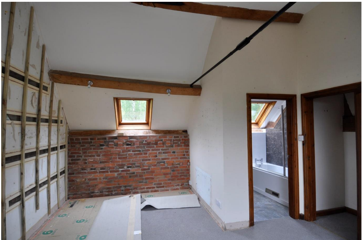
West bedroom looking north
