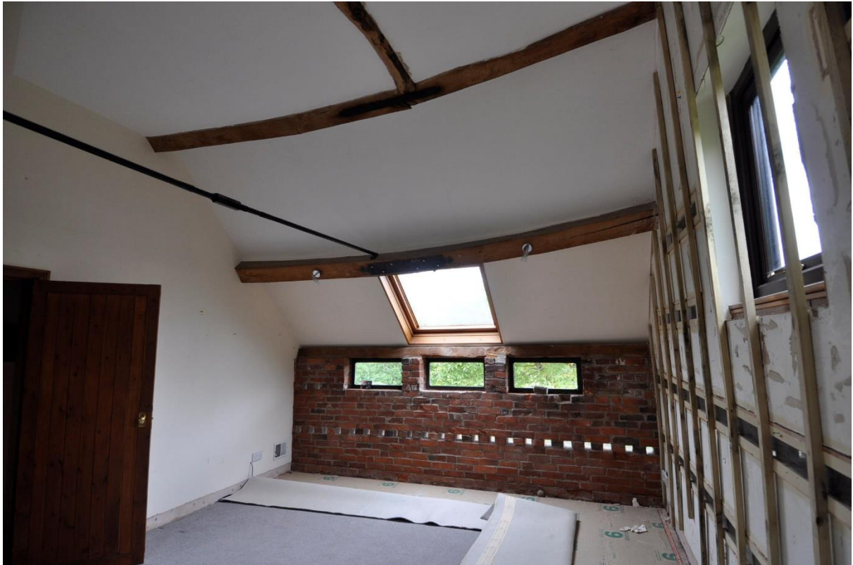
West bedroom looking south
