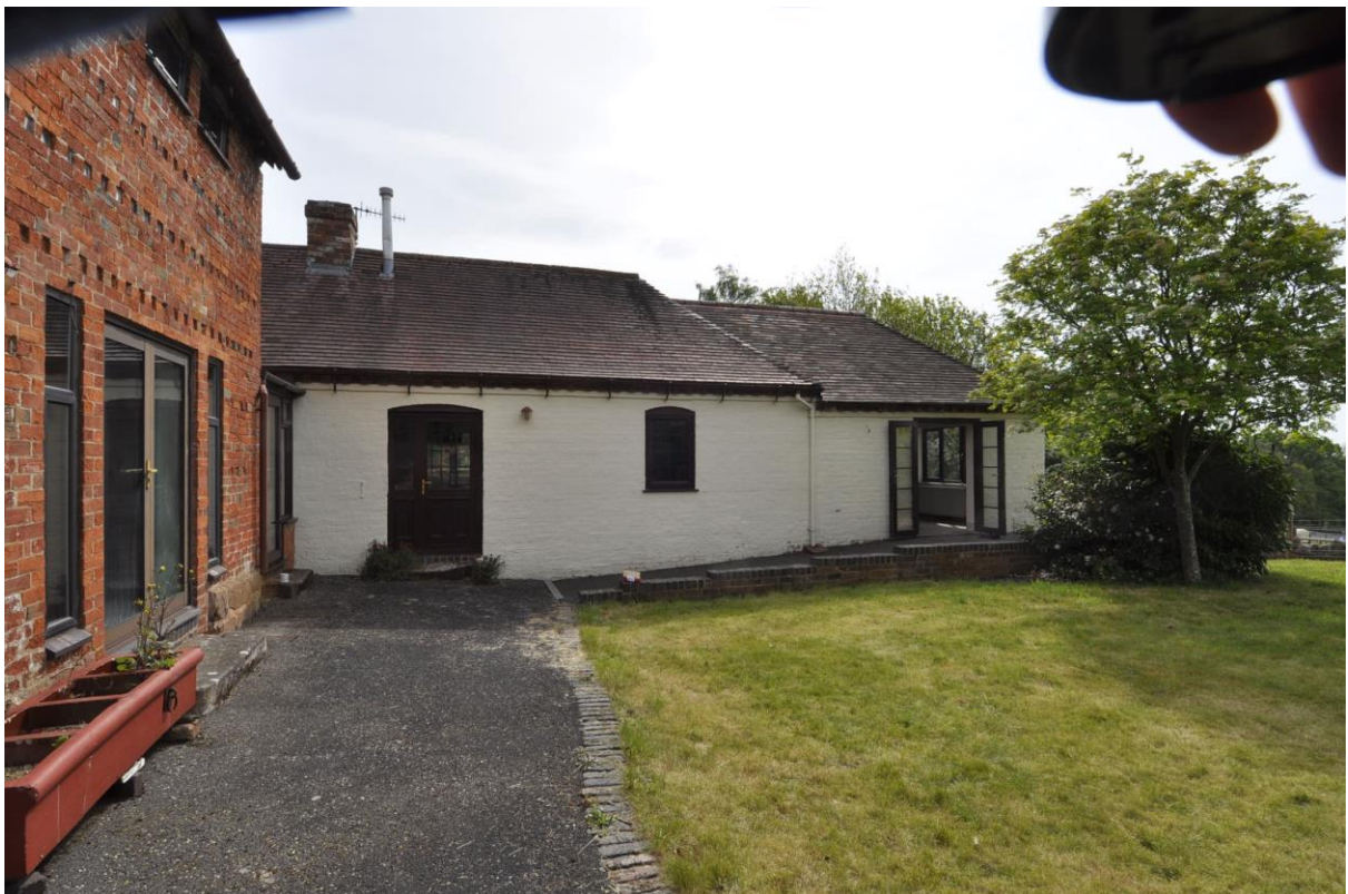
West elevation of wing building
