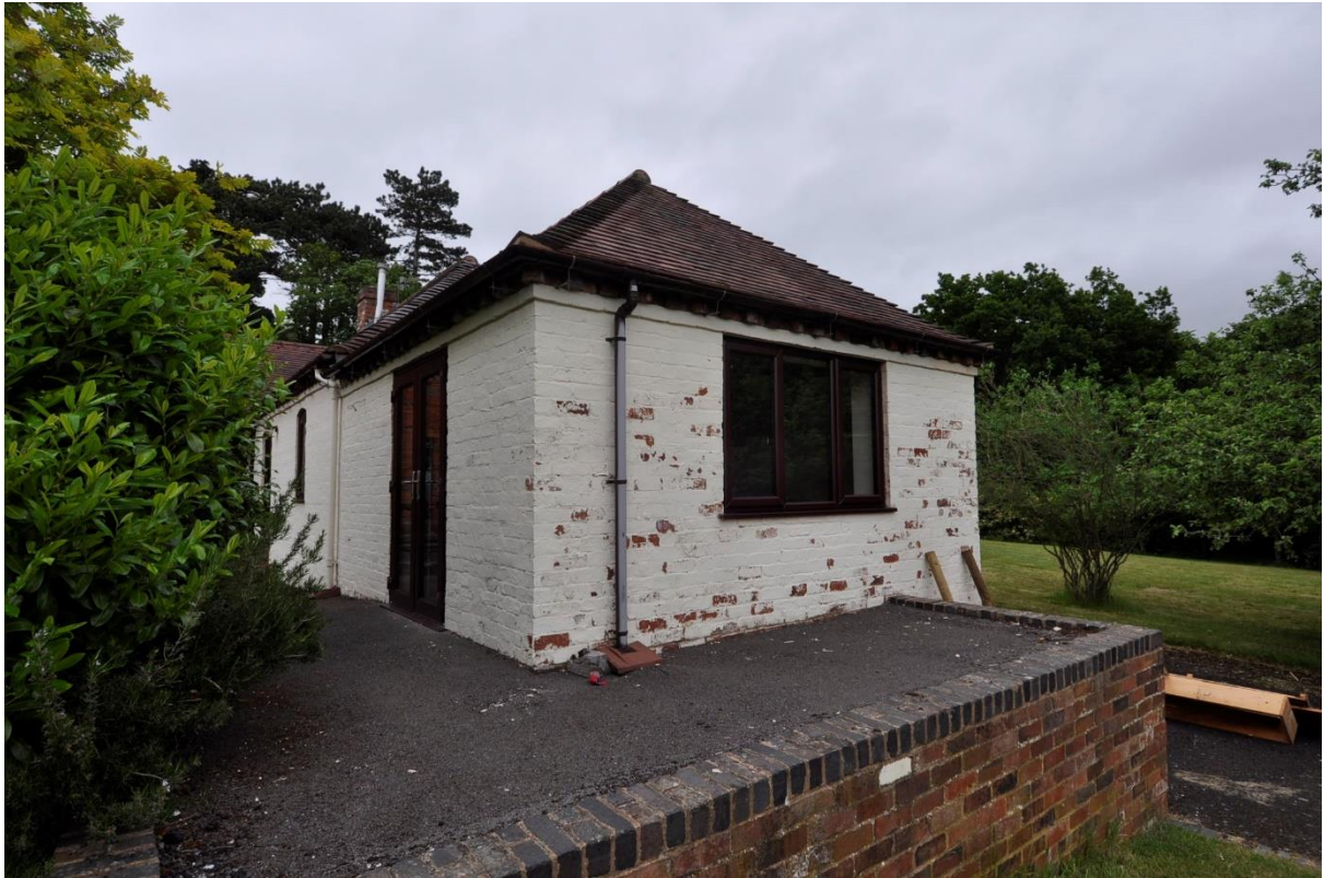
South elevation of wing building
