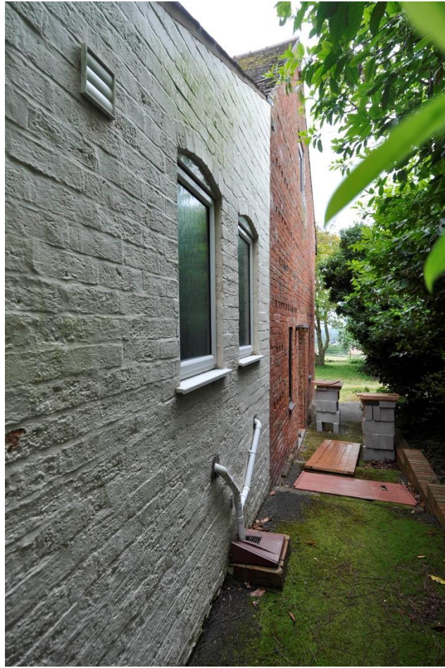
Part west elevation looking south
