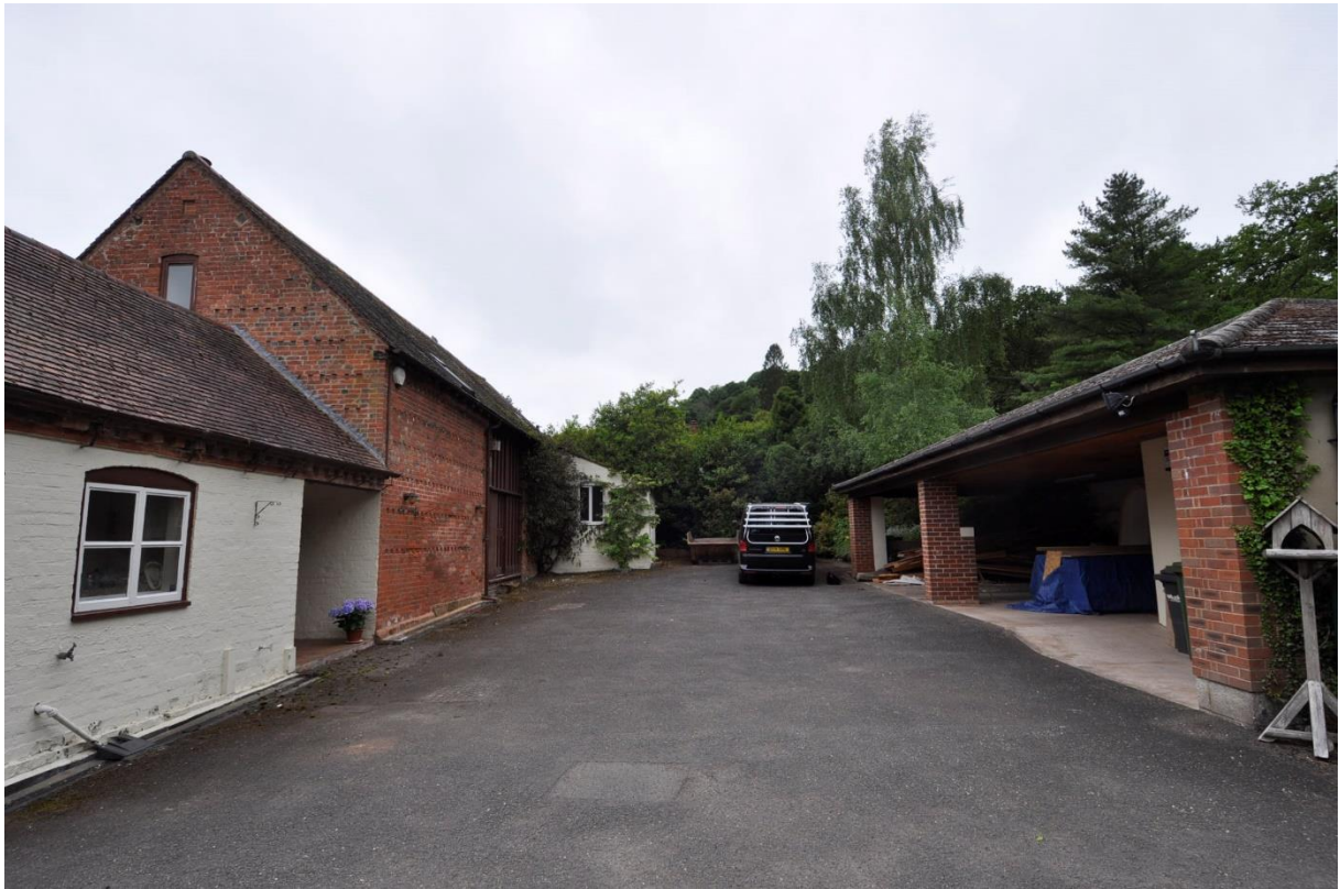
North elevation with carport
