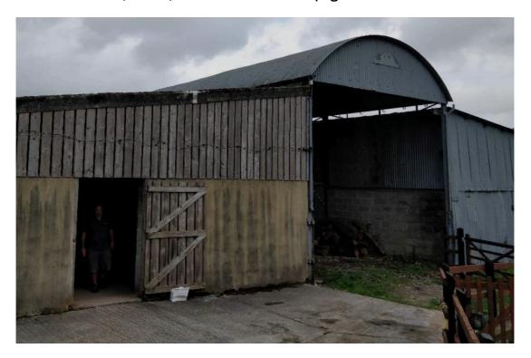
5.1. The section on page 28 shows the building to have a steel frame and cladding. The frame was set in an existing foundation. A new slab floor was proposed along with internal insulation to the walls and roof. The photographs (pages 24 and 25) and plans (26 and 27) showed considerable in-filling of external walls. The Inspector concluded (paragraphs 8 and 9, page 30):
