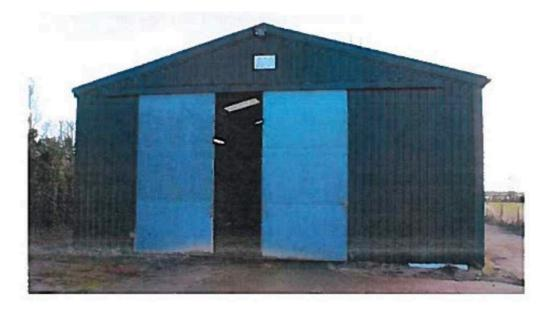
3.1. The building was a steel-clad steel portal frame building with timber purlins and rails and roof bracing. Part of the floor was a concrete slab and the remainder was compacted stone on earth. The cladding was to be retained, a new concrete floor was proposed and insulation was to be added internally. The only external changes were the enlargement of existing openings and the insertion of windows. The
