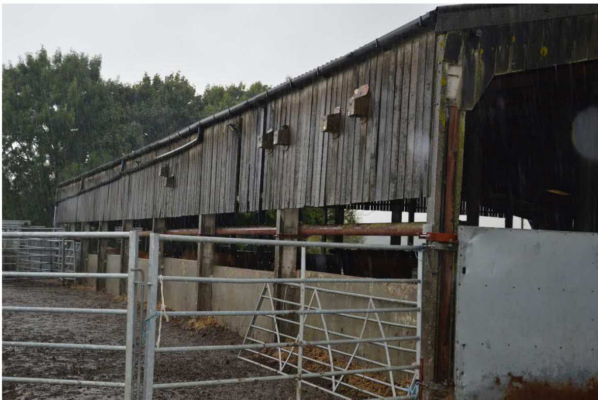
Plate 4. View of east side of the barn 2022.
