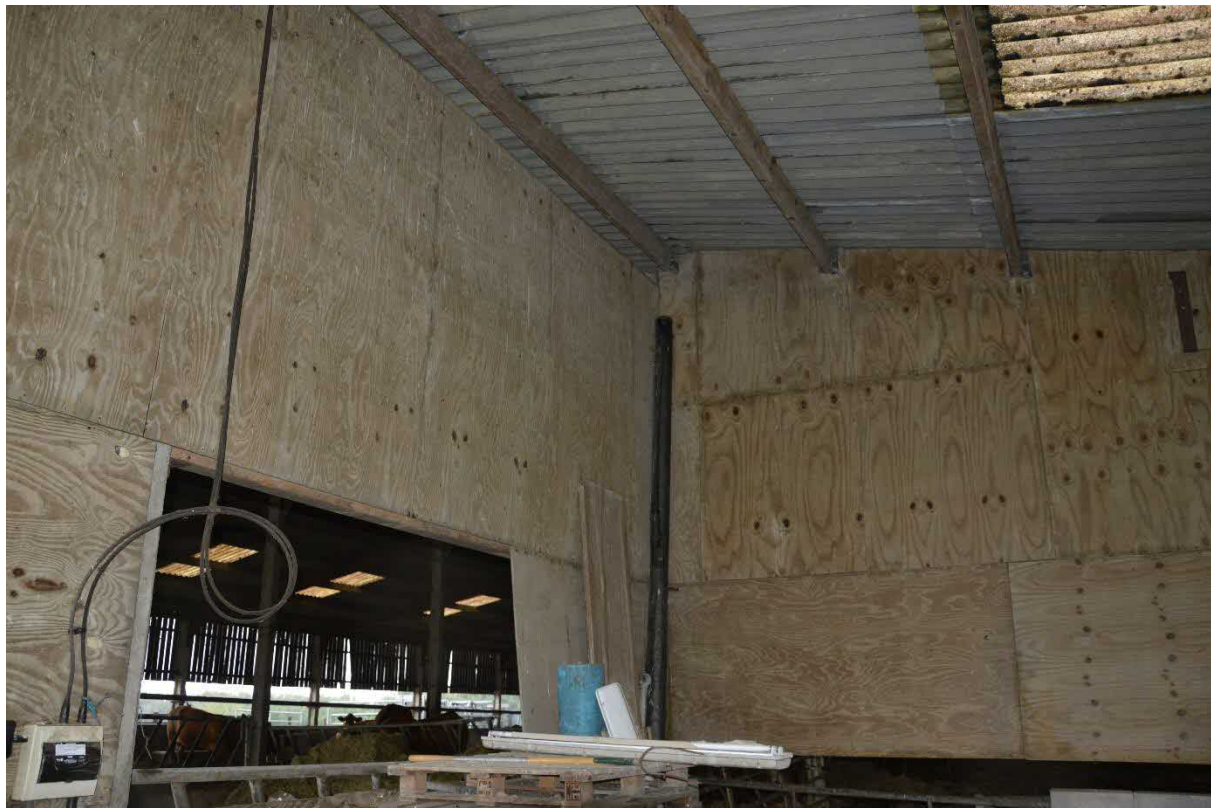
Plate 8. Side section of the barn 2022.
