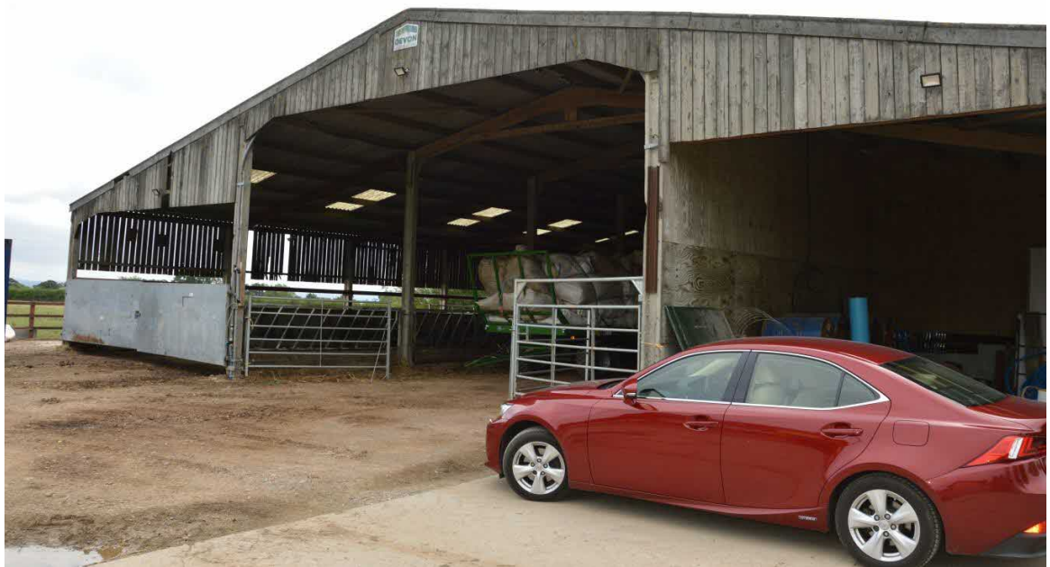
Plate 2. View of barn from the north west 2019.
