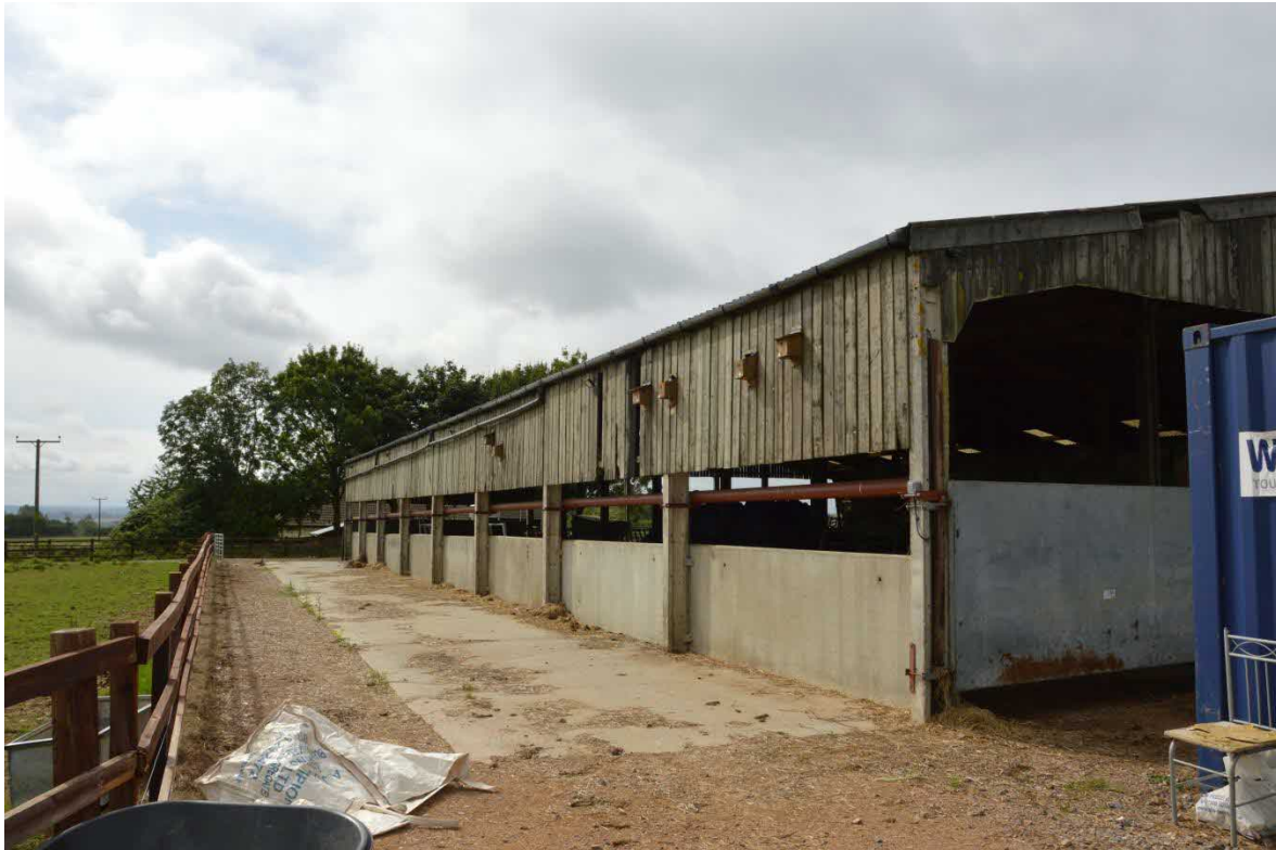
Plate 3. View of east side of the barn 2019.
