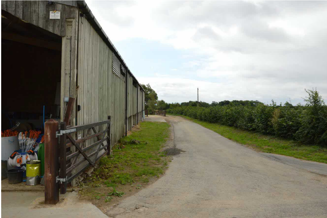
Plate 5. West side of the barn 2019.
