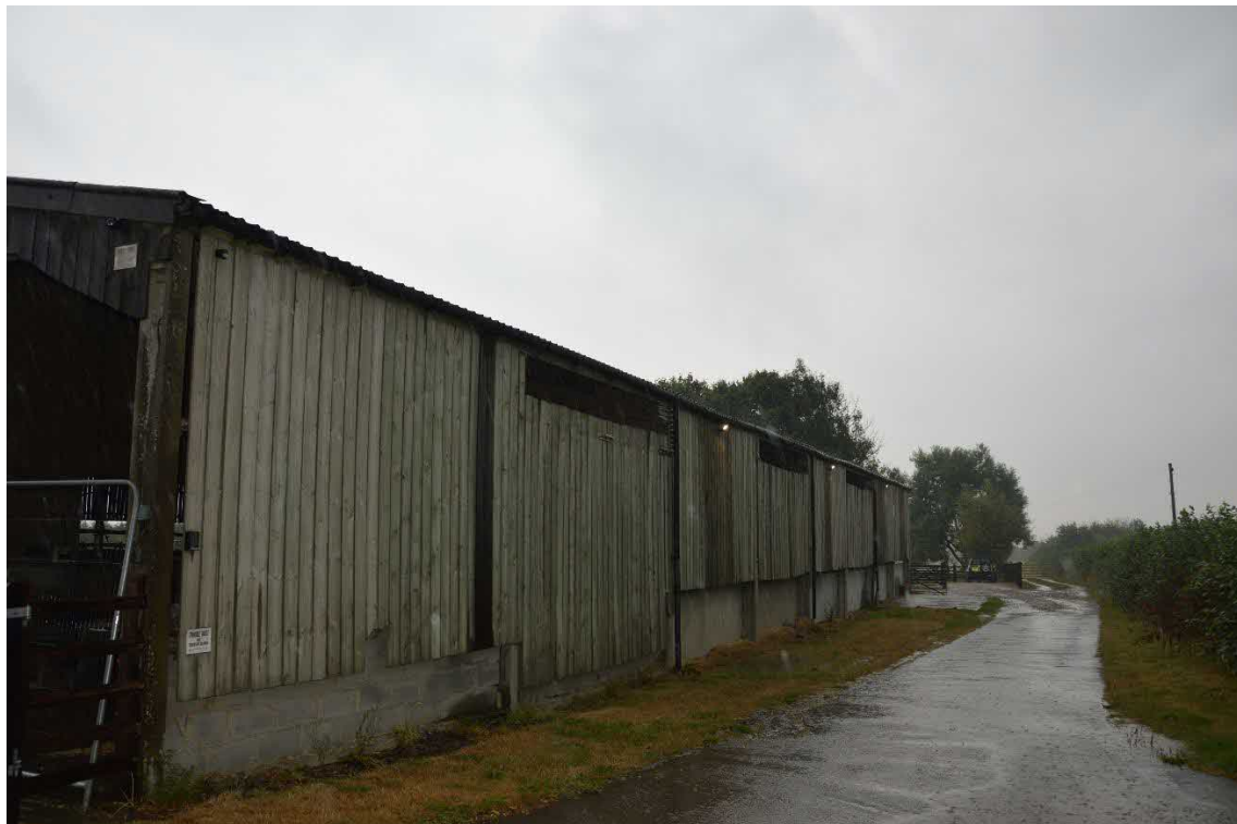
Plate 6. West side of the barn 2022
