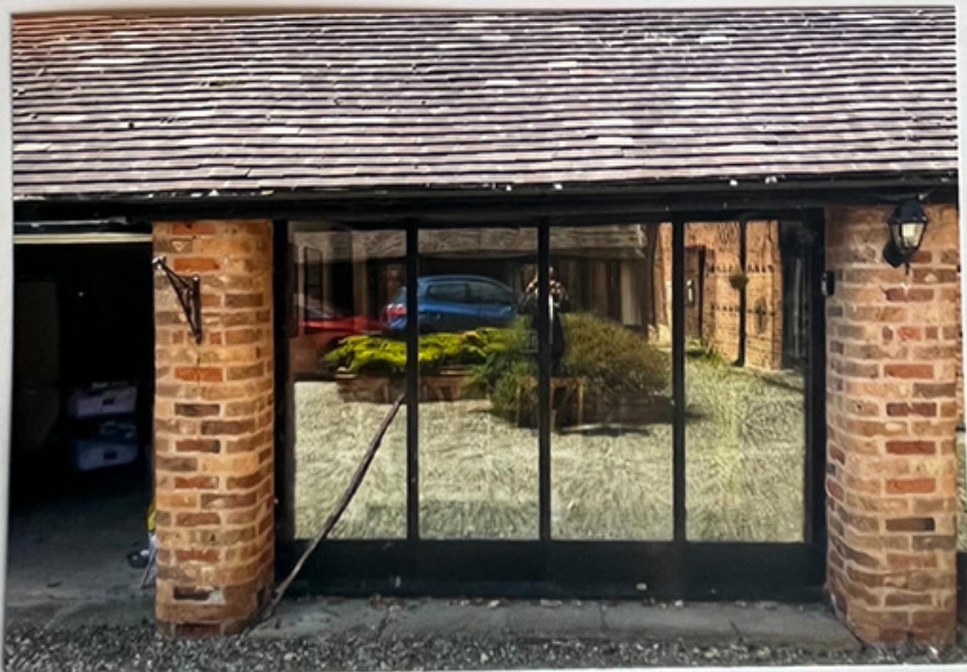
PHOTOGRAPH 7 - DETAIL OF THE ADJOINING BAY WHICH ALREADY HAS A GLAZED SCREEN INSERTED INTO THE FORMER CART SHED OPENING..
