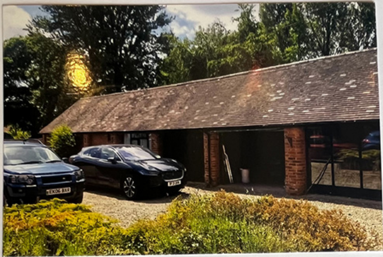
PHOTOGRAPH 4 - DETAIL OF THE COURTYARD SIDE OF THE SINGLE STOREY ROADSIDE RANGE WHICH SHOWS THE FORMER CARTSHED OPENINGS.
