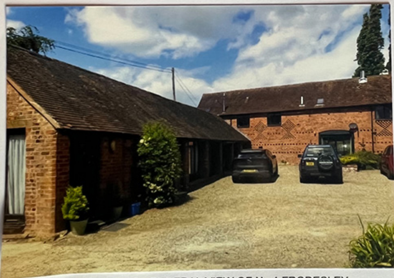
PHOTOGRAPH 3 - GENERAL VIEW OF No.1 FRODESLEY HOUSE FARM BARN AS SEEN FROM THE COURTYARD SIDE.
