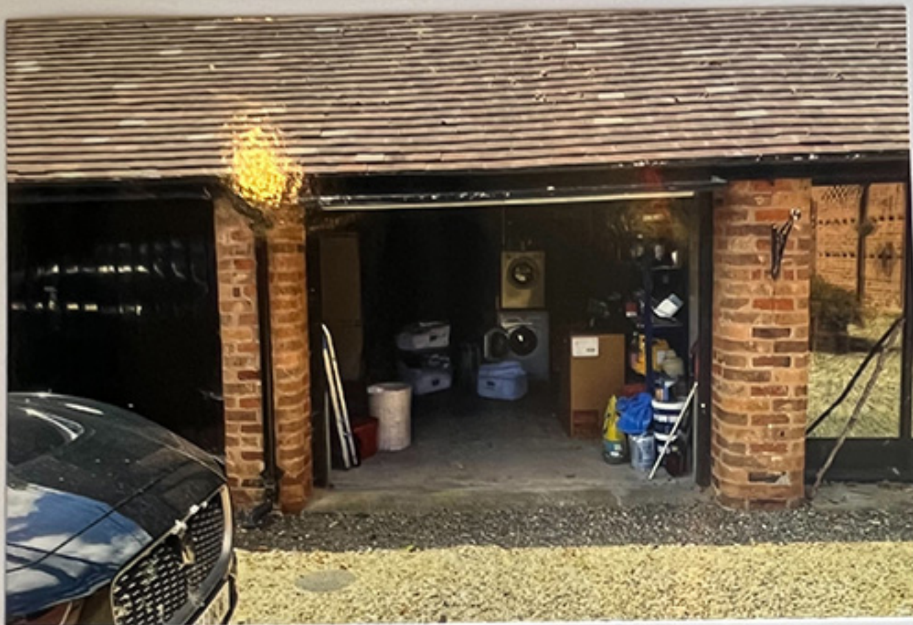
PHOTOGRAPH 6 - DETAIL OF THE EXISTING GARAGE BAY WHICH IT IS PROPOSED TO INCORPORATE AS A UTILITY ROOM. THE GARAGE DOOR WOULD BE REPLACED WITH A GLAZED SCREEN INCORPORATING A WOODEN DOOR.
