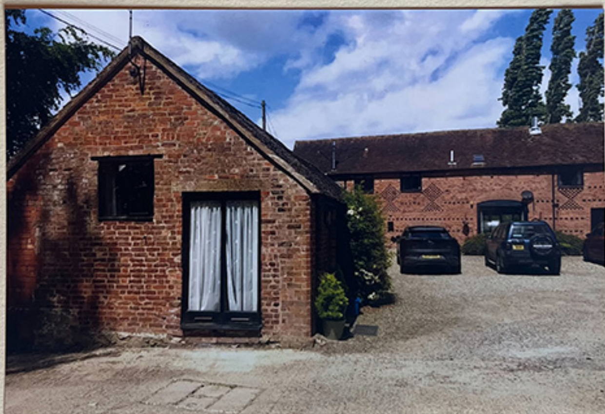
PHOTOGRAPH 1 - GENERAL VIEW OF No.1 FRODESLEY HOUSE FARM BARN.
