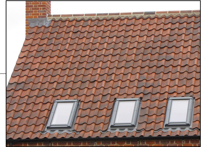
Lifestiles Ashvale Restoration Clay Pantiles to Houses
