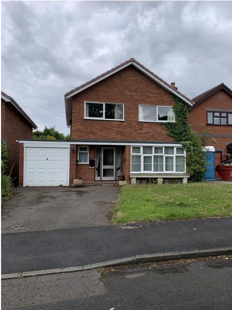
View towards the front of the existing dwelling
