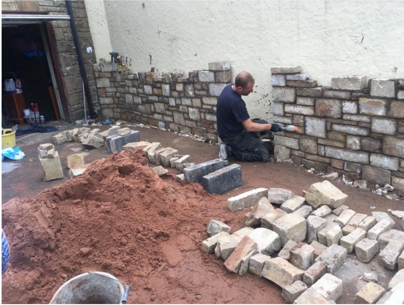
Picture showing new stone facing being applied to existing render wall.
