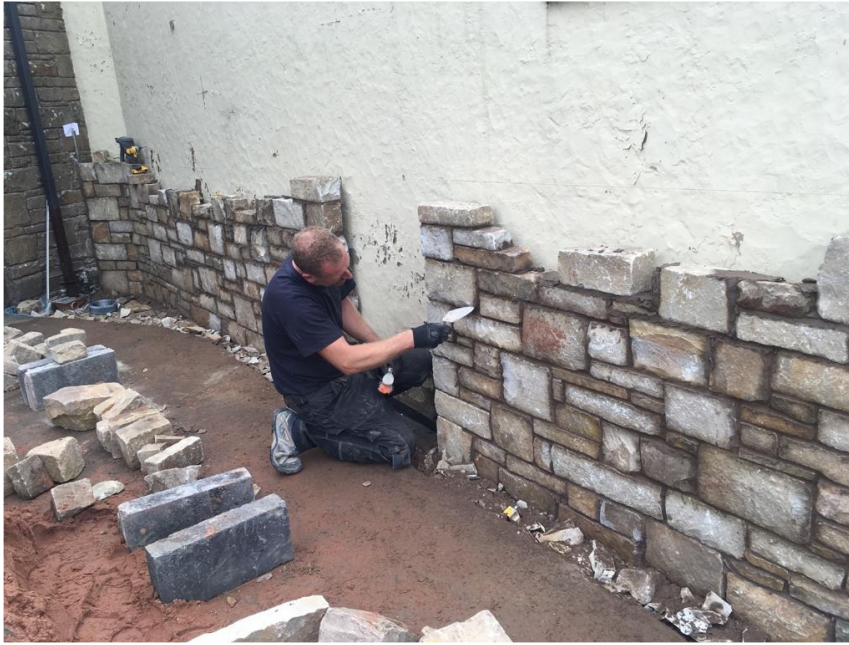
Picture showing existing rendered wall being faced.
