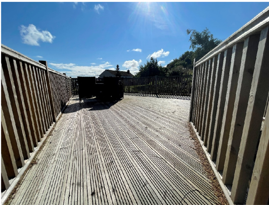
Picture from decking looking south east commenced June 2021 completed Aug 2021
