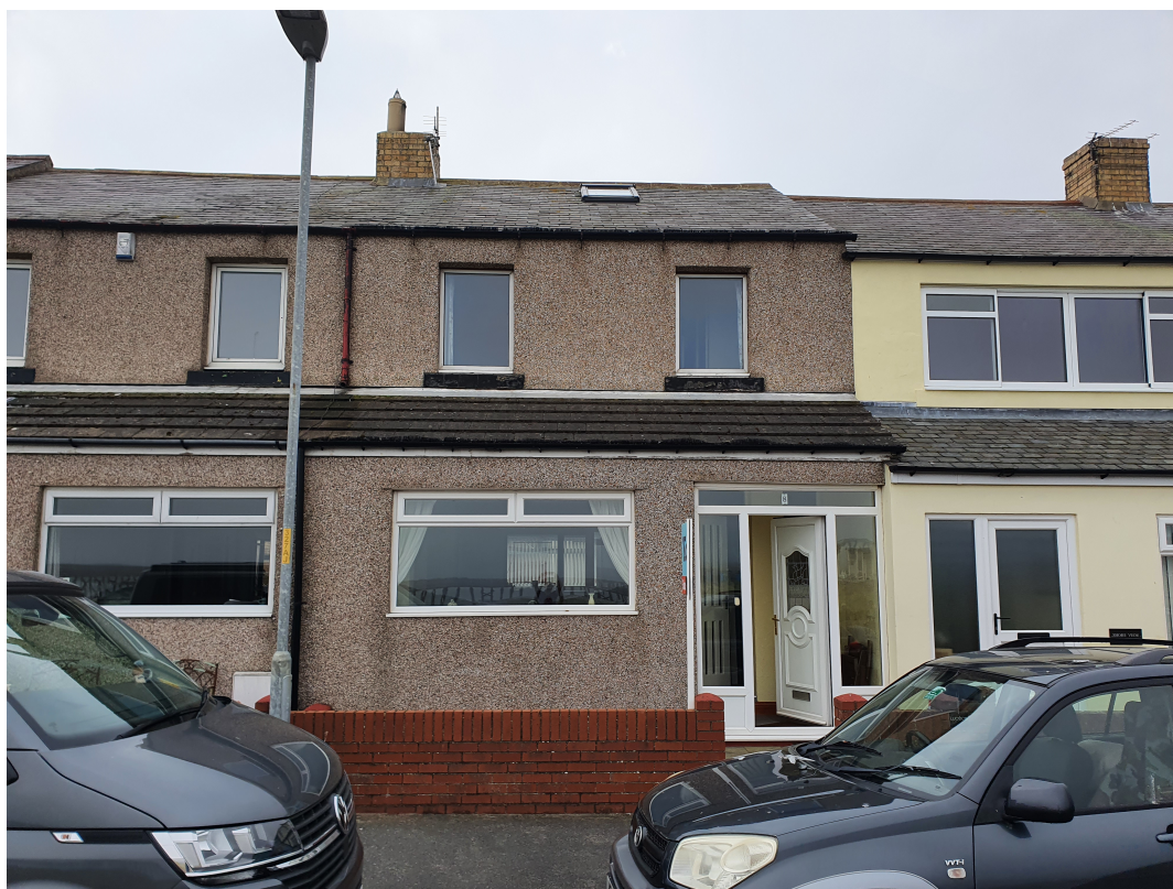
Photo: Existing North Elevation
