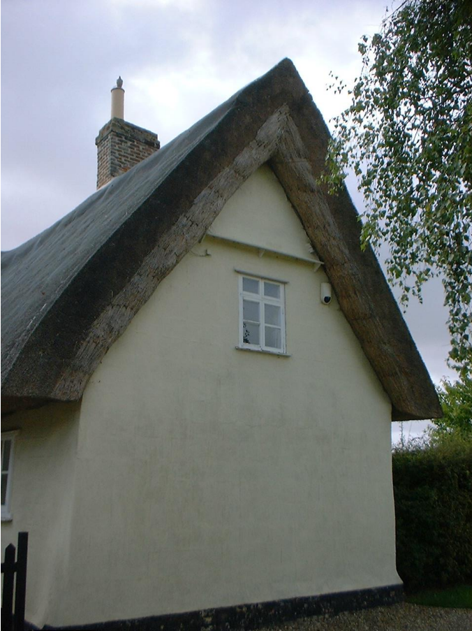
West gable end
