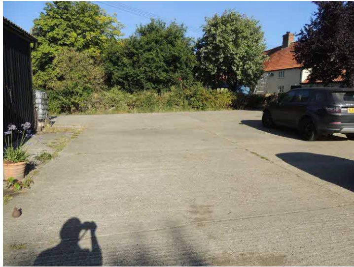
Photo 14: Looking eastwards from the barn. Note extent of hardstanding
