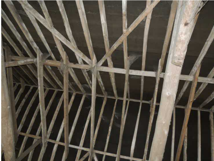
Photo 5: Showing roof structure
