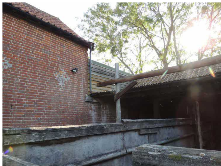
Photo 6: Outbuilding to the south-east
