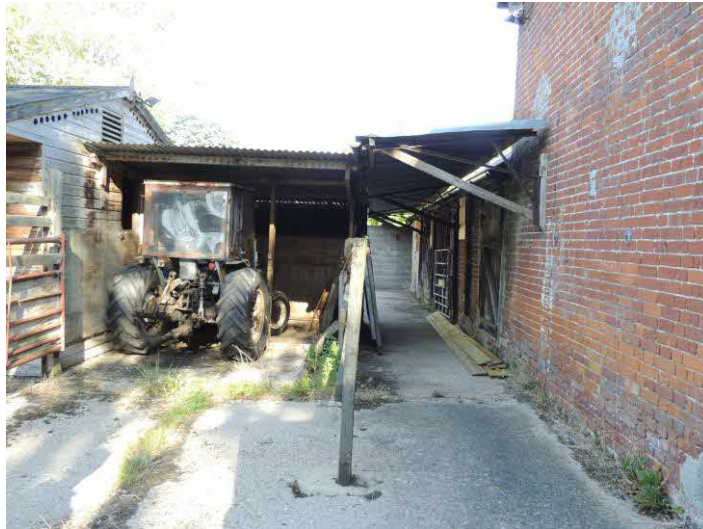
Photo 8: Two lean-tos on the southern side are to be demolished
