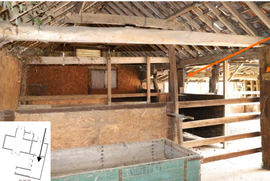
Fig. 29: East shelter shed looking south with its two original posts for west open front
