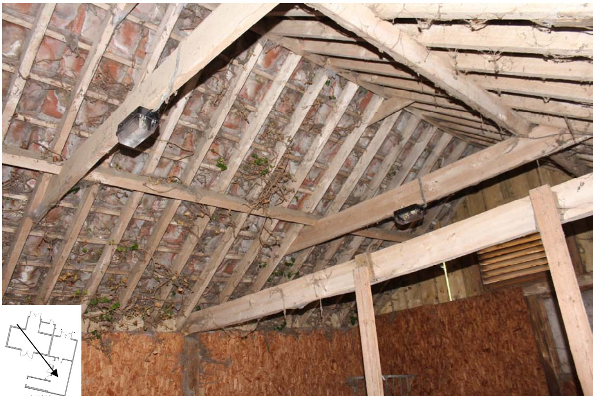
Fig. 27 Roof of east shelter shed looking south-east
