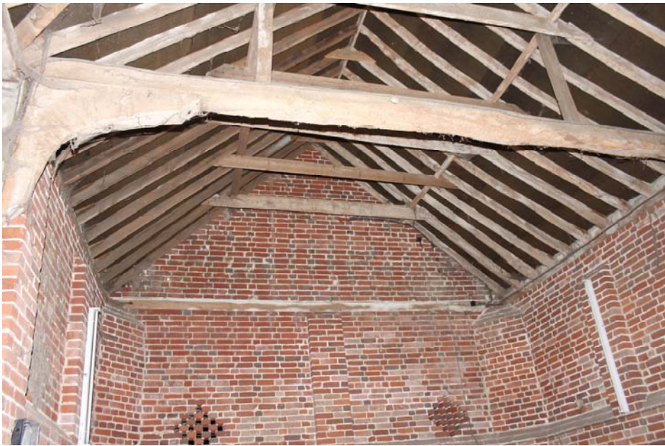
Fig. 8: Roof of barn looking west
