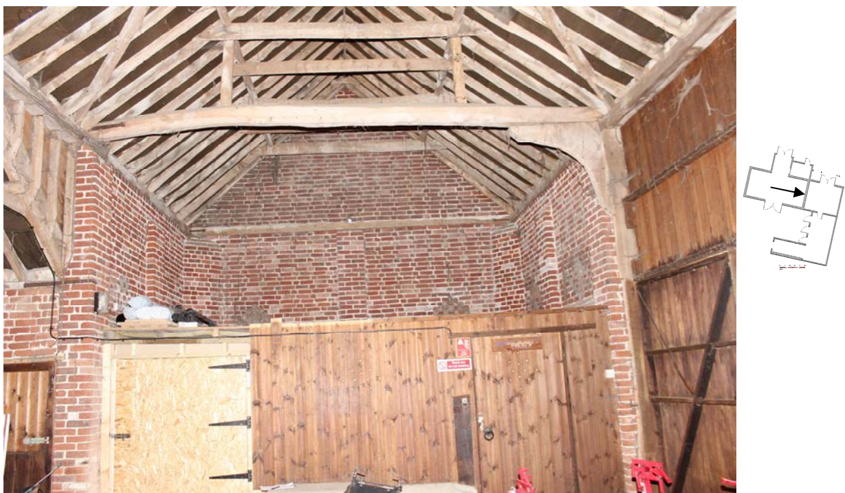
Fig. 7: East half of barn showing tiebeam with knee brace only at south end. Loft is a later insertion
