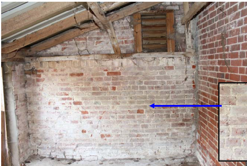
Fig. 21: East wall of lean-to shed on east side of midstrey is built in a mixed bond
