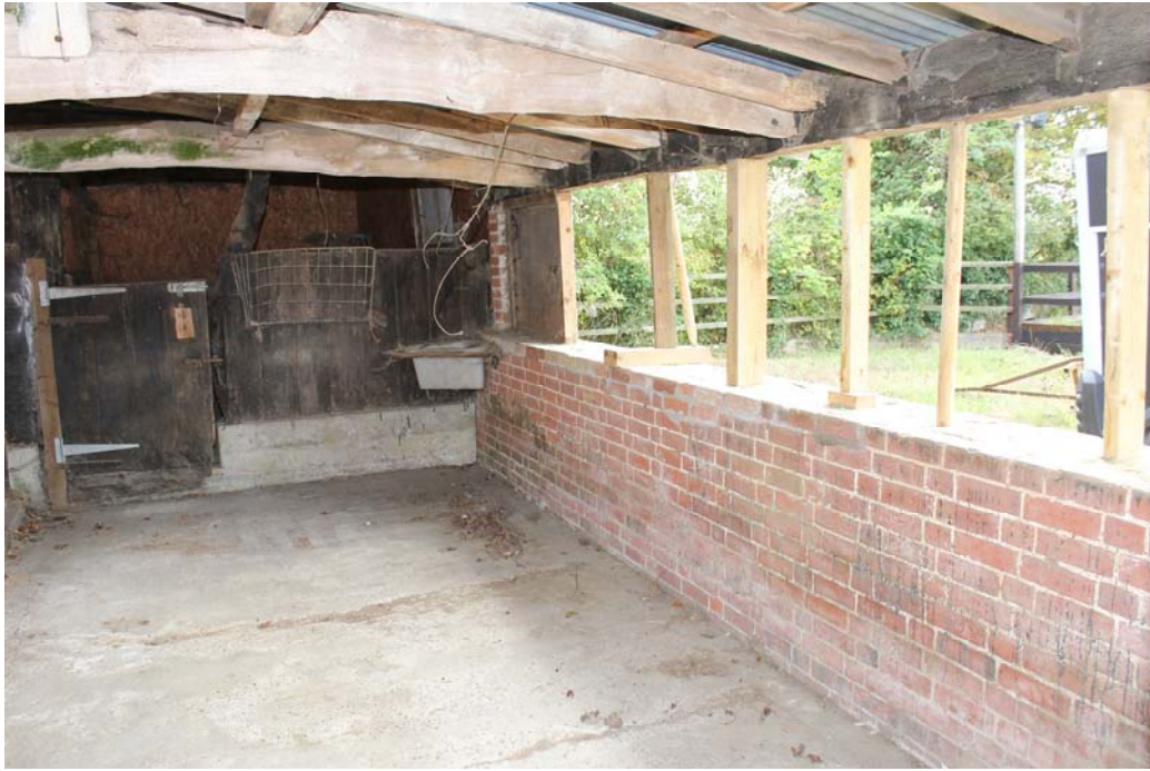
Fig. 35: Interior of bottom of 'L' shelter shed looking east
