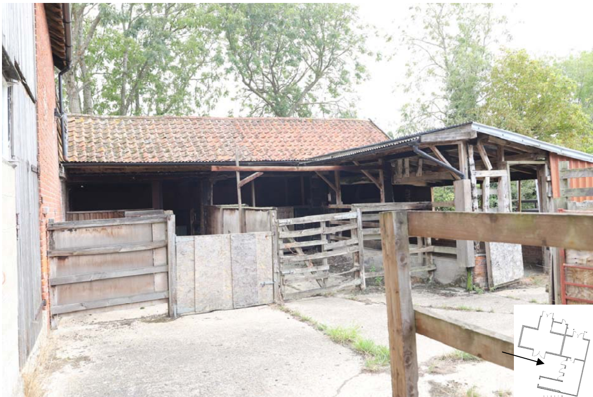
Fig. 23: Cattle yard looking east
