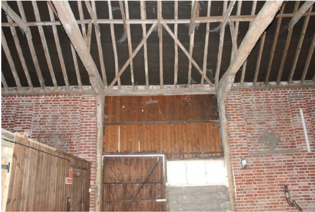
Fig. 11: South end of threshing bay where the large full height doors have been replaced
