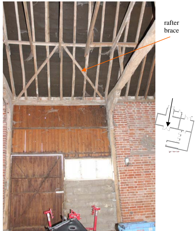
Fig. 6: Rafter bracing south end of threshing bay
