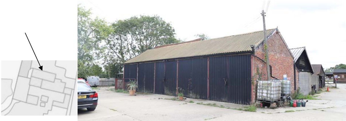
Fig. 17: North front of large building which replaced the lost west lean-to shed
