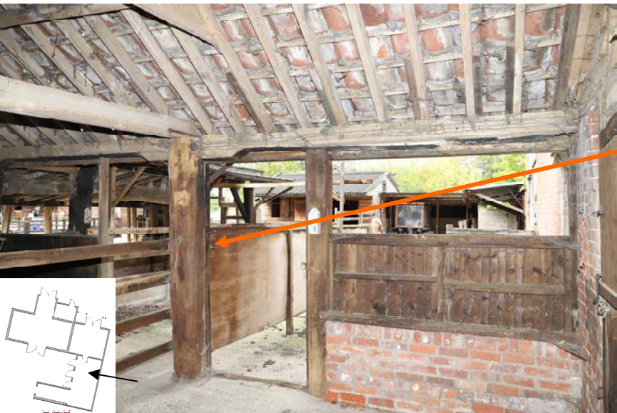
Fig. 30: West wall of shelter shed with northern original post highlighted
