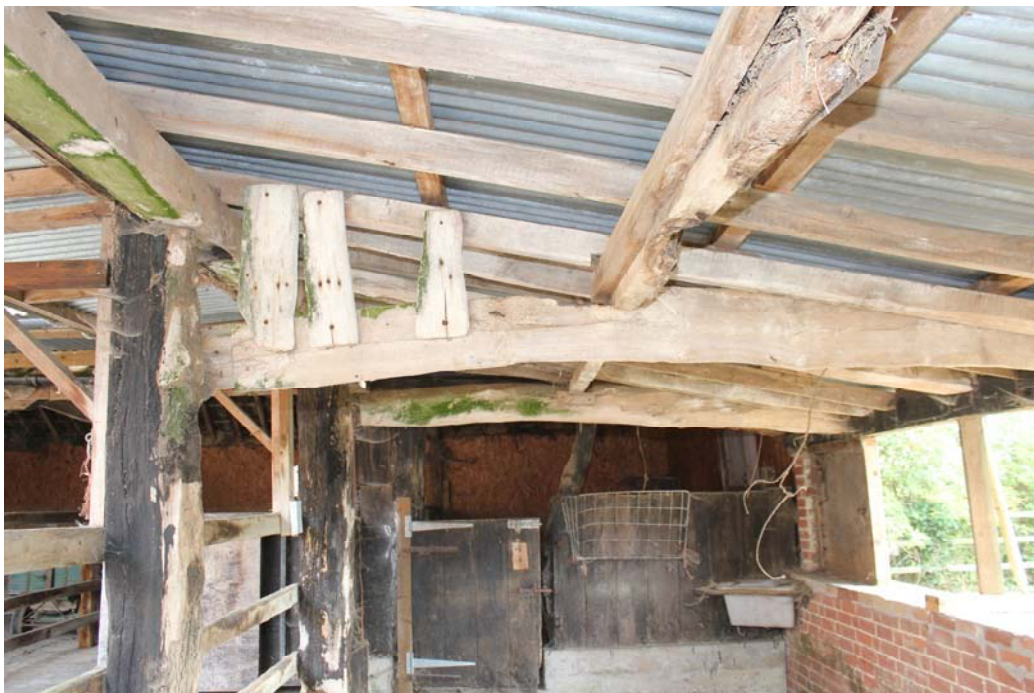
Fig. 36: Roof of bottom of 'L' shelter shed looking east
