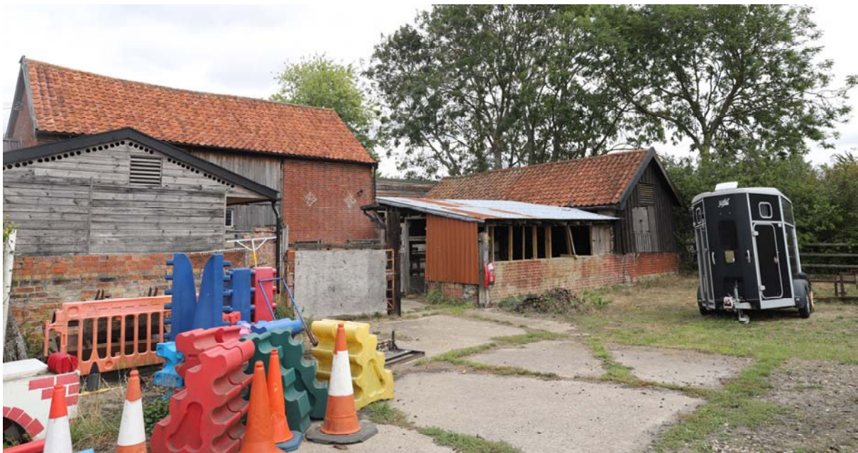
Fig. 4: South side of barn
