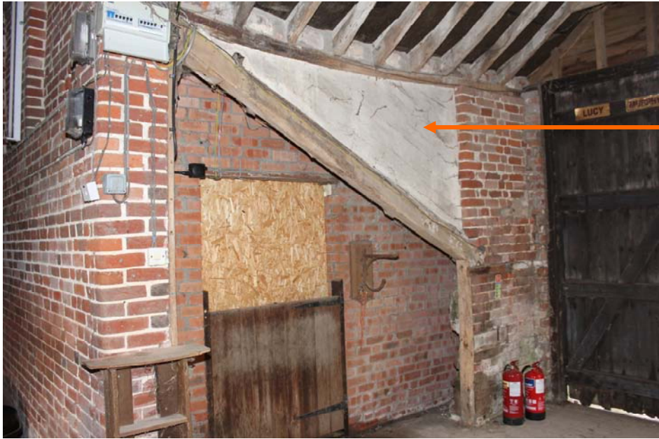
Fig. 16: West wall of midstrey incorporating end wall of lost west lean-to shed
