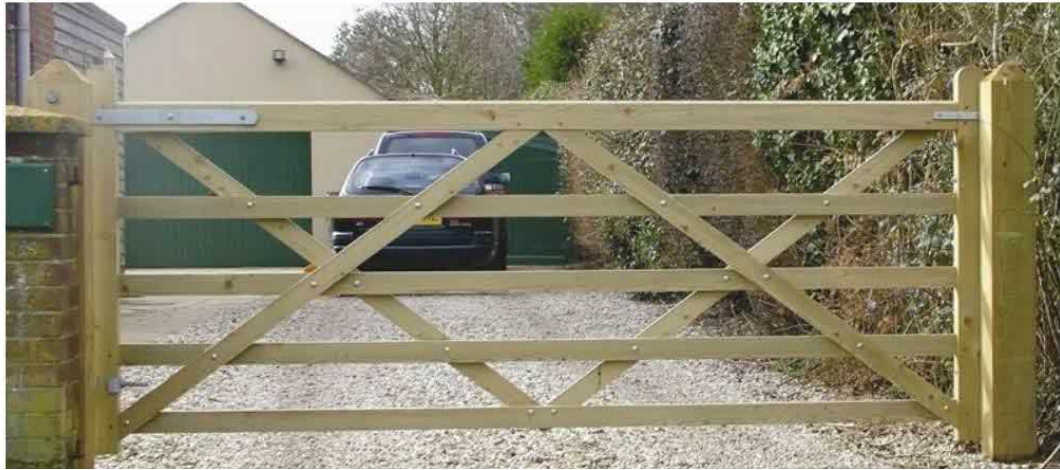
Figure 2: 5-bar timber gate
