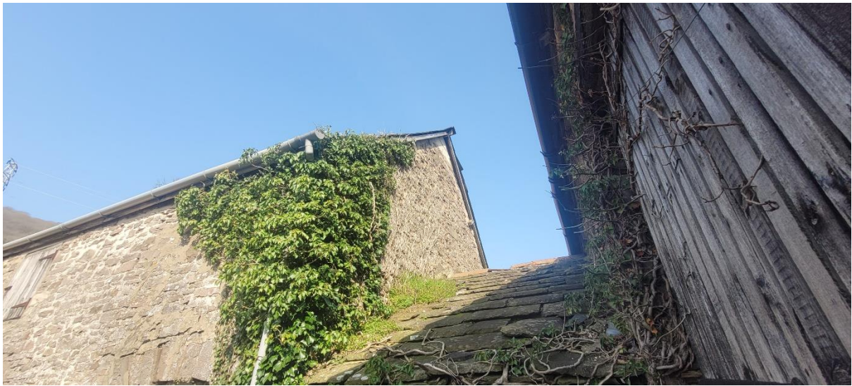
Plate 7 – link building (southern elevation) & Building 2 eastern gable end
