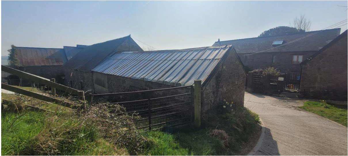
Plate 3 – Buildings 1 & 2 rear (northern) and side (western) elevations
