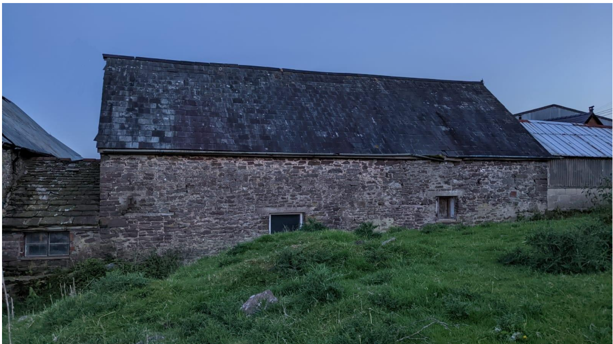
Plate 8 – Link building & Building 2 rear (northern) elevation
