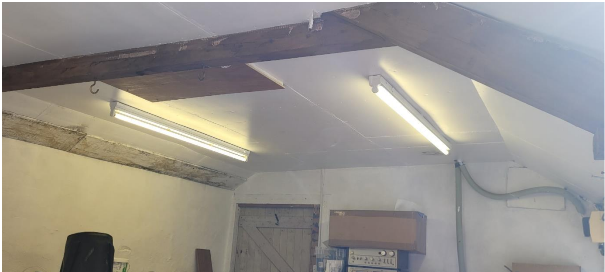
Plate 4 – Building 1 internal view
