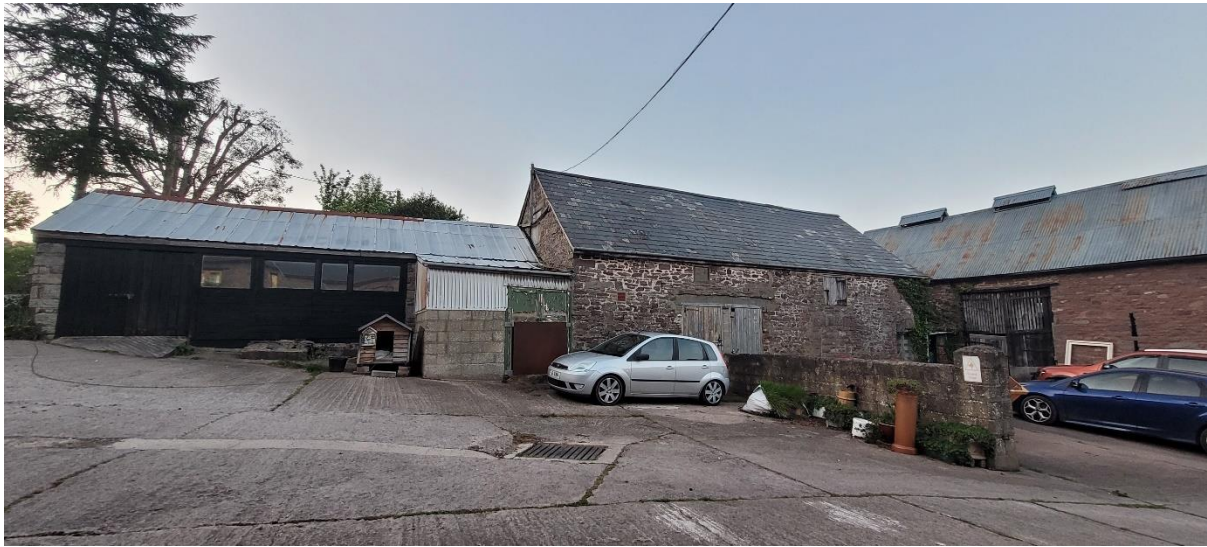
Plate 1 – Buildings 1 & 2 front (southern) elevation
